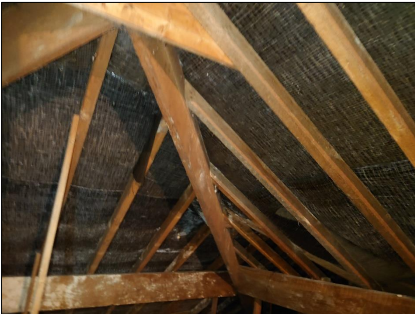
Photograph 14 showing the roof lining and timbers
