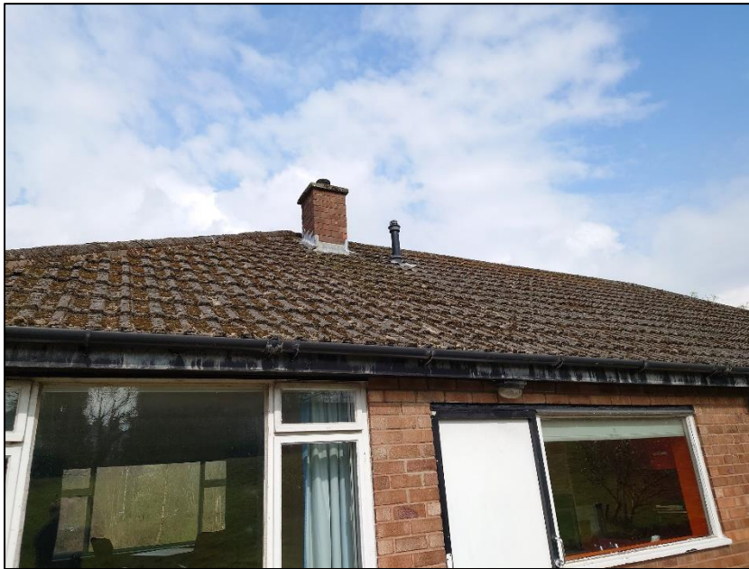
Photograph 11 showing the roof of the bungalow
