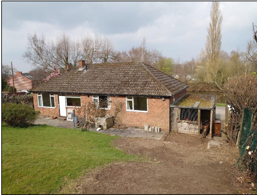
Photograph 9 showing the rear of the dwelling
