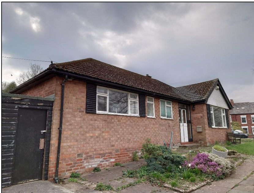
Photograph 8 showing the front of the dwelling
