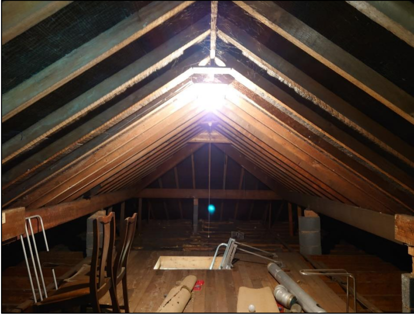
Photograph 13 showing the roof void
