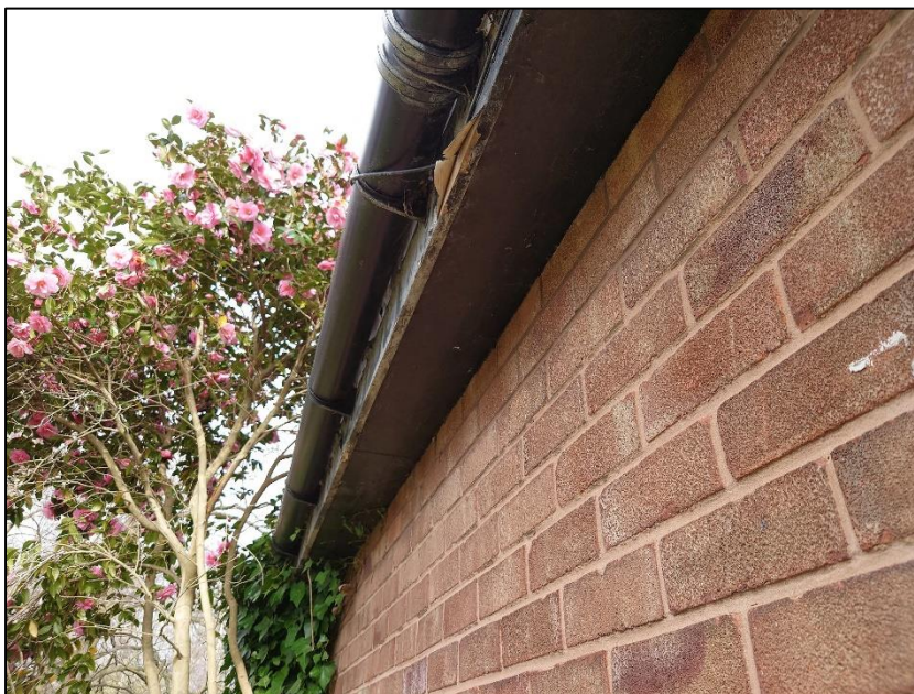
Photograph 12 showing the soffits and bargeboards
