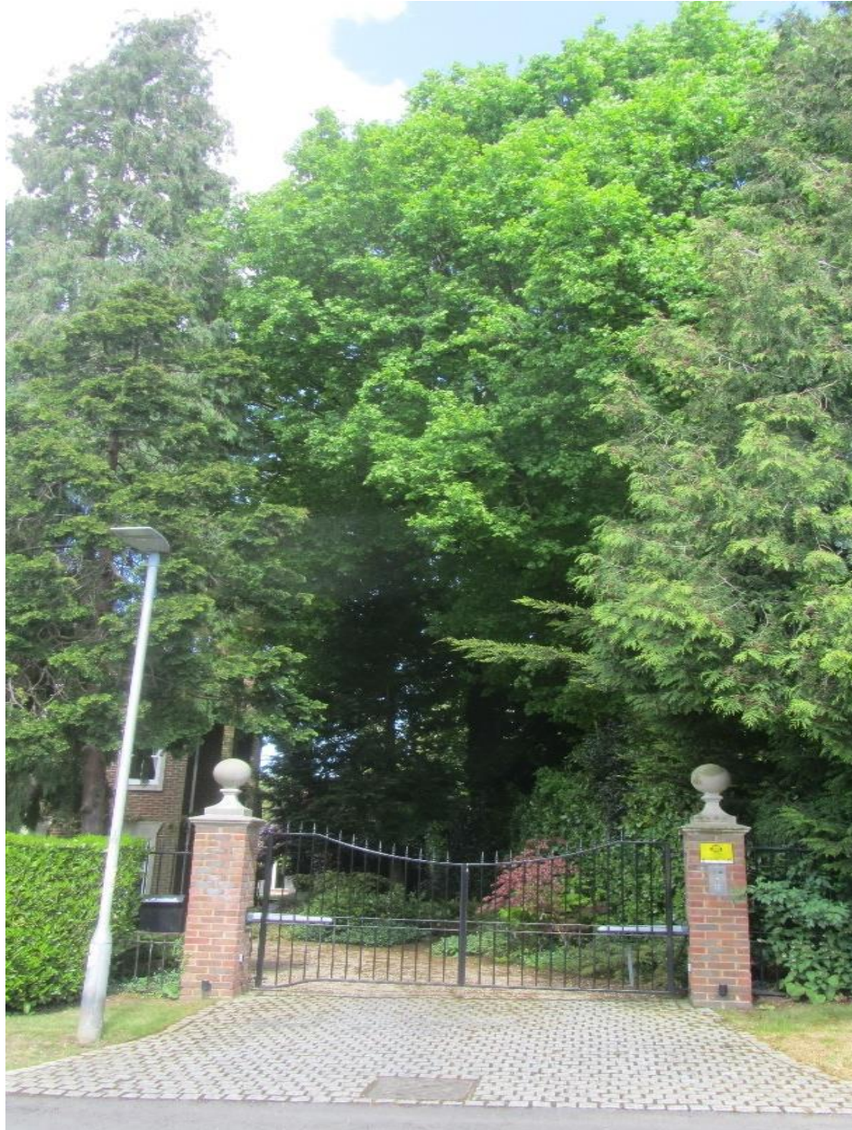
PHOTOGRAPH NO. 4 – T13 & T14 SHOWING CROWNS GROWING OVER THE DRIVEWAY AND DWELLING HOUSE OF NO. 30 THE AVENUE
