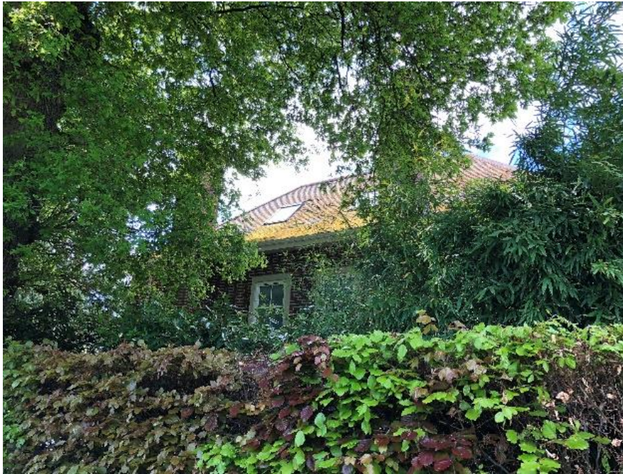
PHOTOGRAPH NO. 8 – LATERAL BRANCHES OF T13 & T14 ENCROACHING INTO THE CURTILAGE OF NO. 30 THE AVENUE
