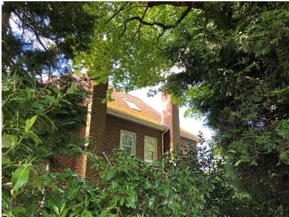
PHOTOGRAPH NO. 7 – LATERAL BRANCHES OF T13 & T14 ENCROACHING INTO THE CURTILAGE OF NO. 30 THE AVENUE
