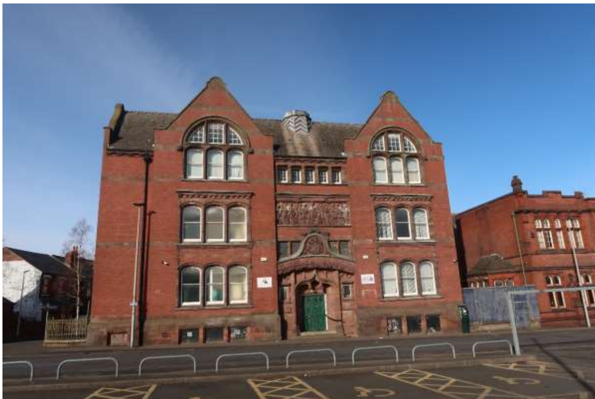
Figure 33: Principal elevation of the Ryland Memorial School of Art
