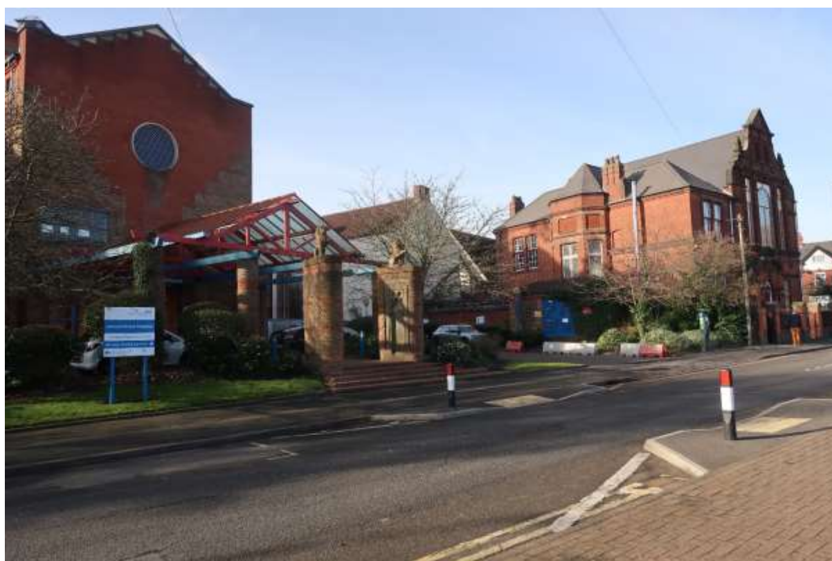
Figure 39: Westerly view from Edward Street with only glimpse views of the rear of the church
