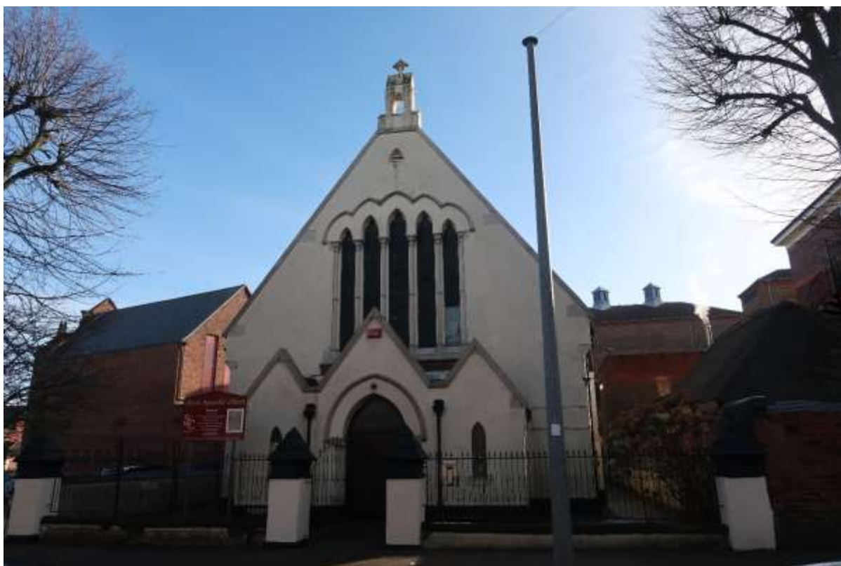
Figure 38: Principal elevation of the Shiloh Apostolic Church
