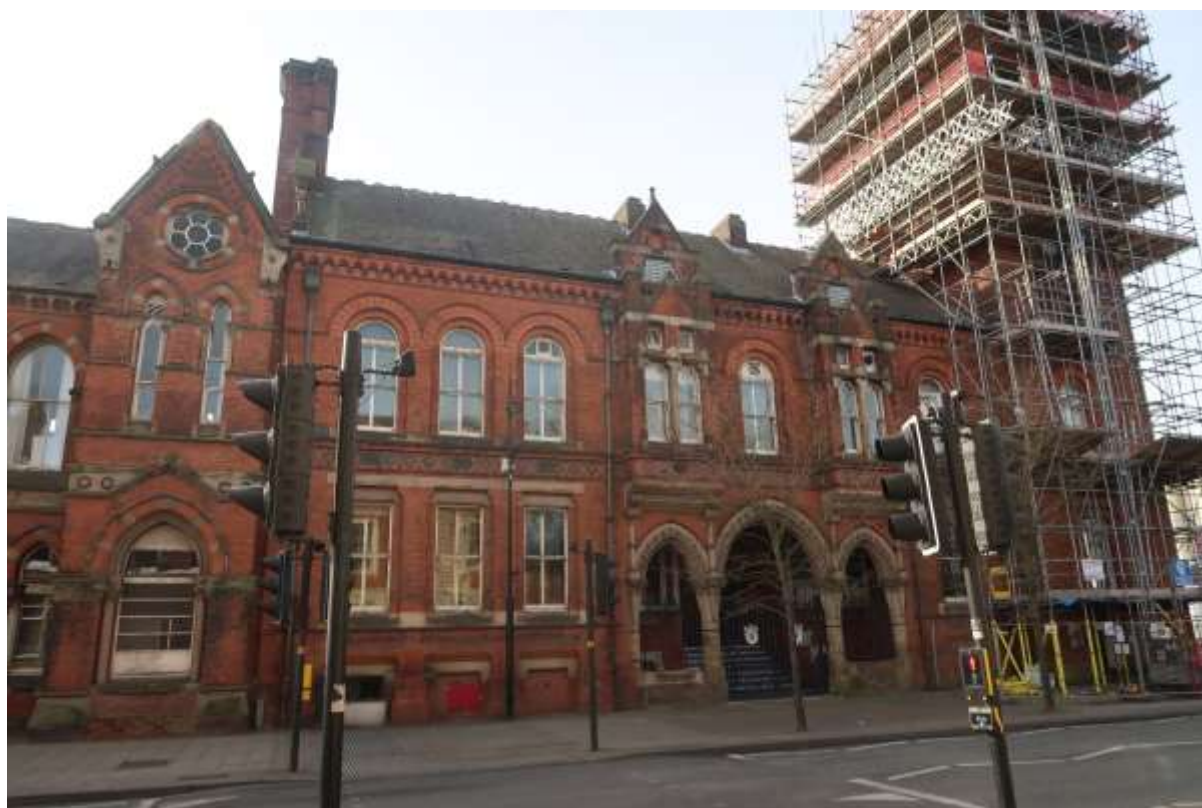
Figure 24: Principal elevation of the Town Hall
