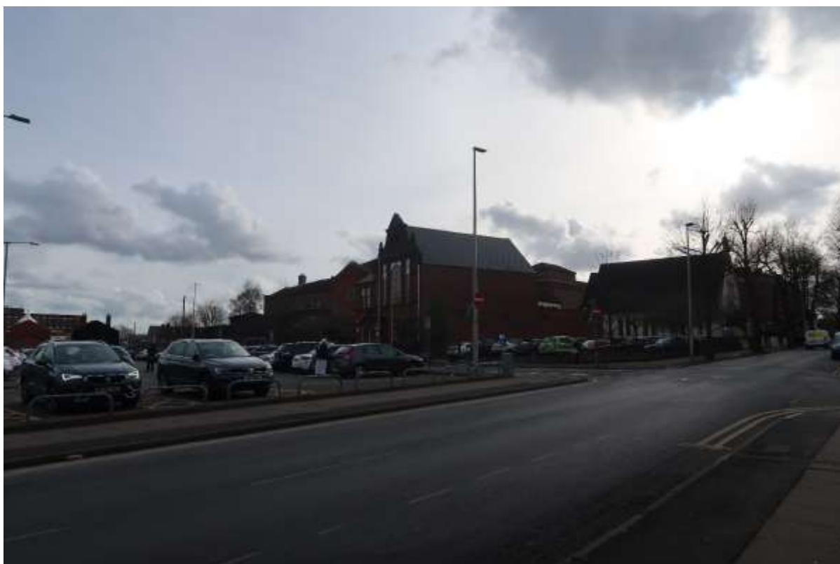
Figure 37: View of the Site and Masonic Hall along Edward Street
