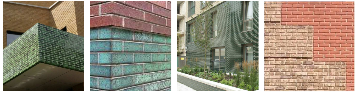
EDWARD ST HOSPITAL EXISTING FAÇADE - DETAIL
