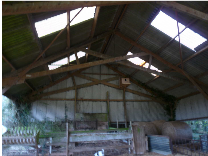
Photo 5: Looking SE within the barn
