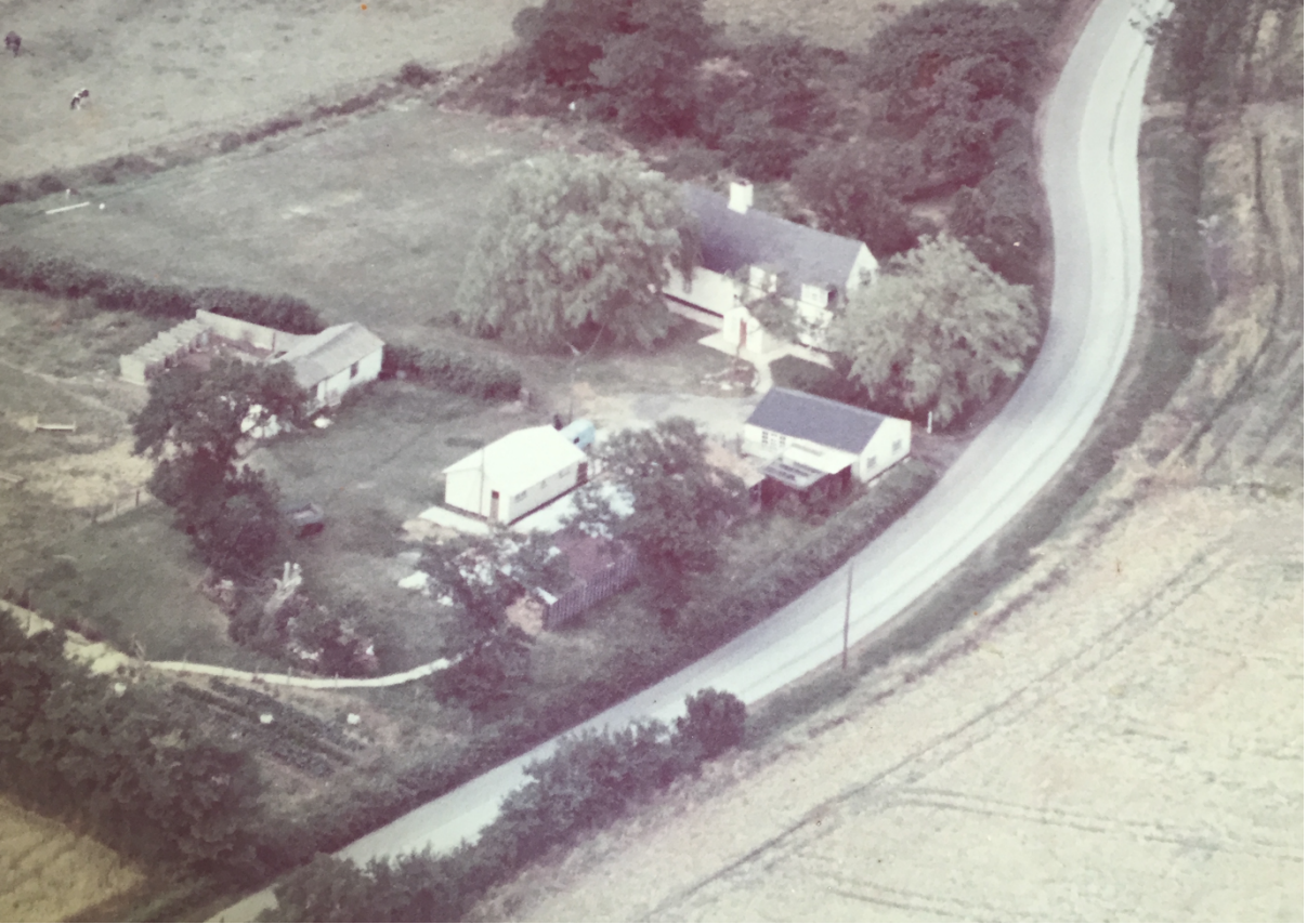
Site Photo from the 1960s
