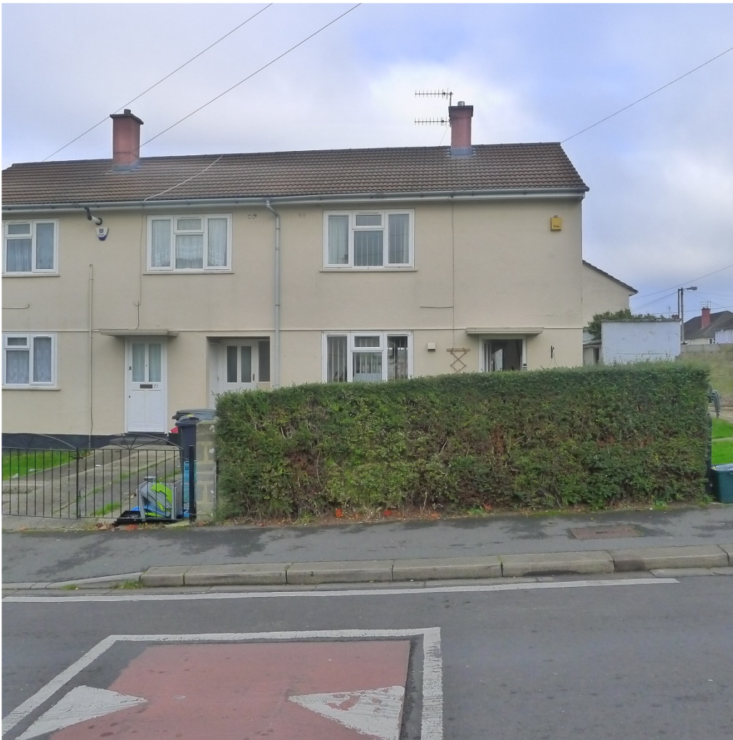
Front Elevation of No. 79
