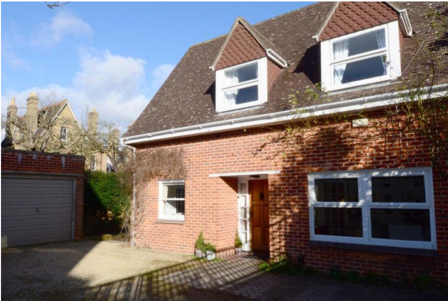
Existing red brick and terracotta tiled/ clad house with gable dormer windows facing South West
