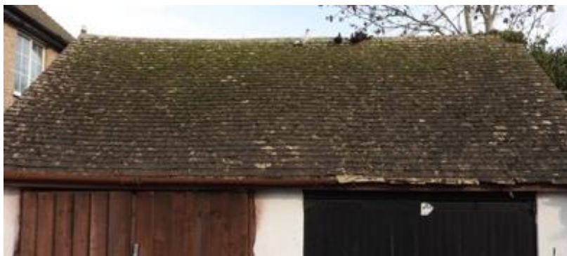
Fig. 25 Ridge and roof tiles on the west side
