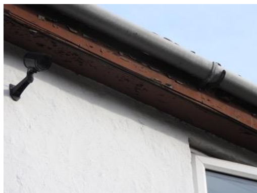
Figs. 23 & 24 Sealed eaves – house (L) and flat roofs (R)
