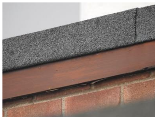
Figs. 23 & 24 Sealed eaves – house (L) and flat roofs (R)
