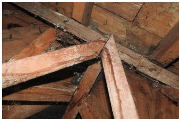
Fig. 14 Cobwebbed plumb cut
