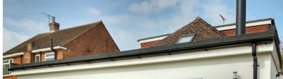
IMAGE 6: BLACK METAL PARAPET TO PERIMETER OF EXTENSION
