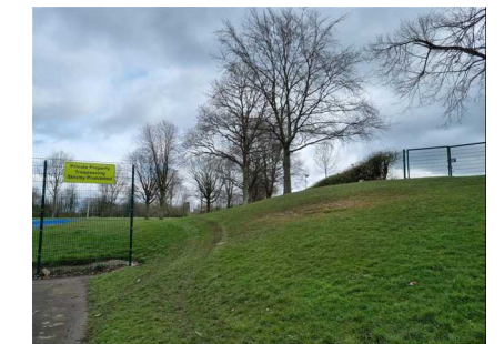
Extend existing fence to meet fence at the top of the bank
