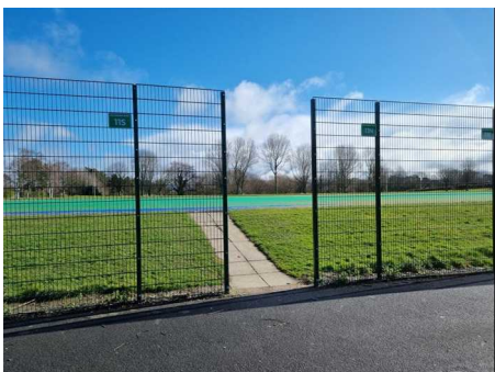
Existing Photo Gate 3A & Gate 3B
