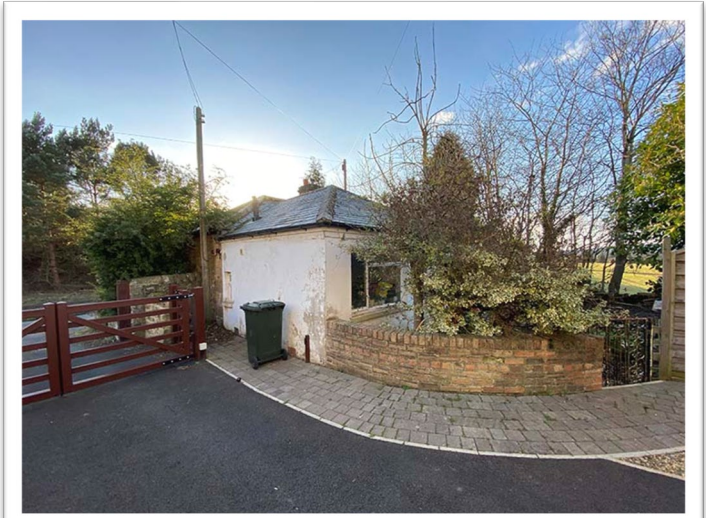
Figure 6 Showing the east and north elevation of the 1950s flat-roof extension to which a pitch was subsequently added
