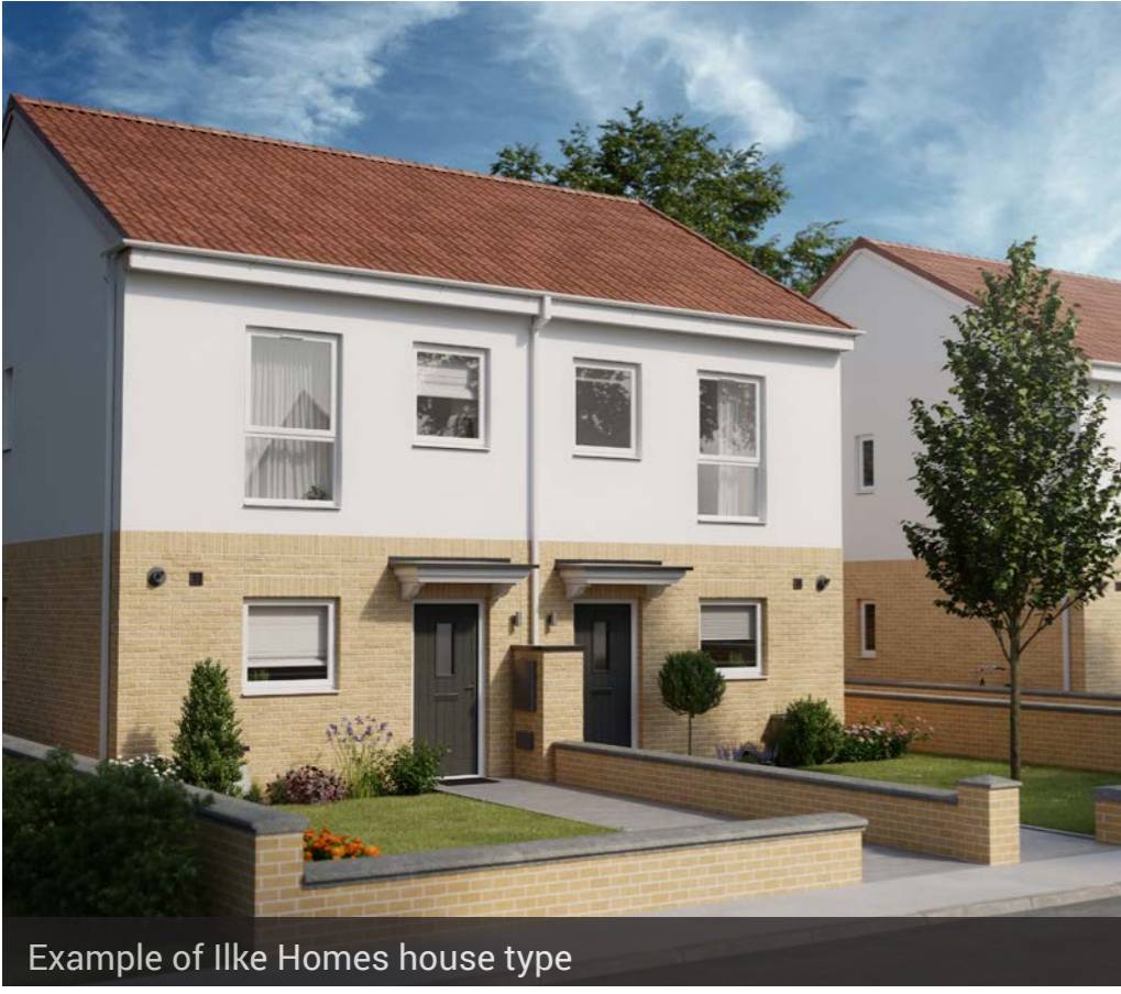
Example of Ilke Homes house type
