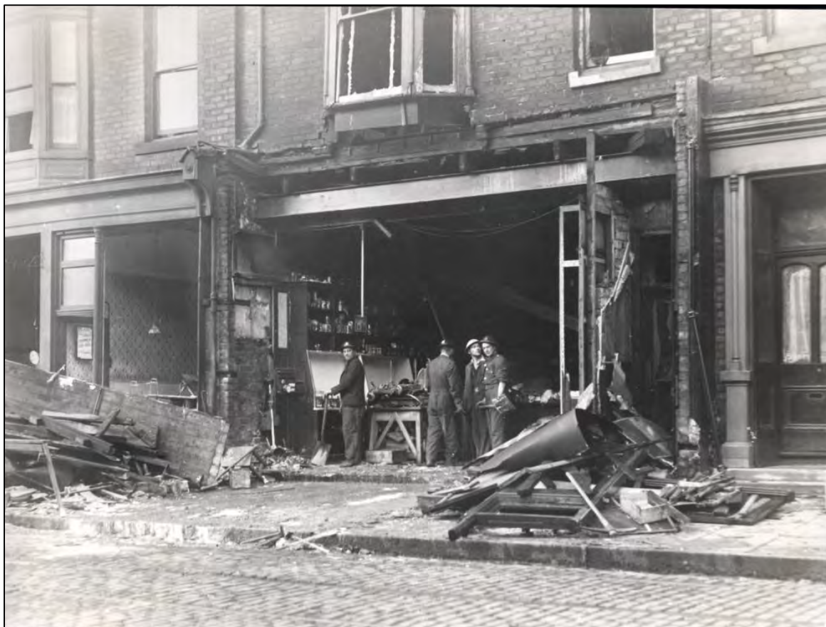
Above: 23.15 hrs 5th September 1940 Front of 55 ½ Suffolk street, showing result of fire after German aircraft had crashed in the backyard
