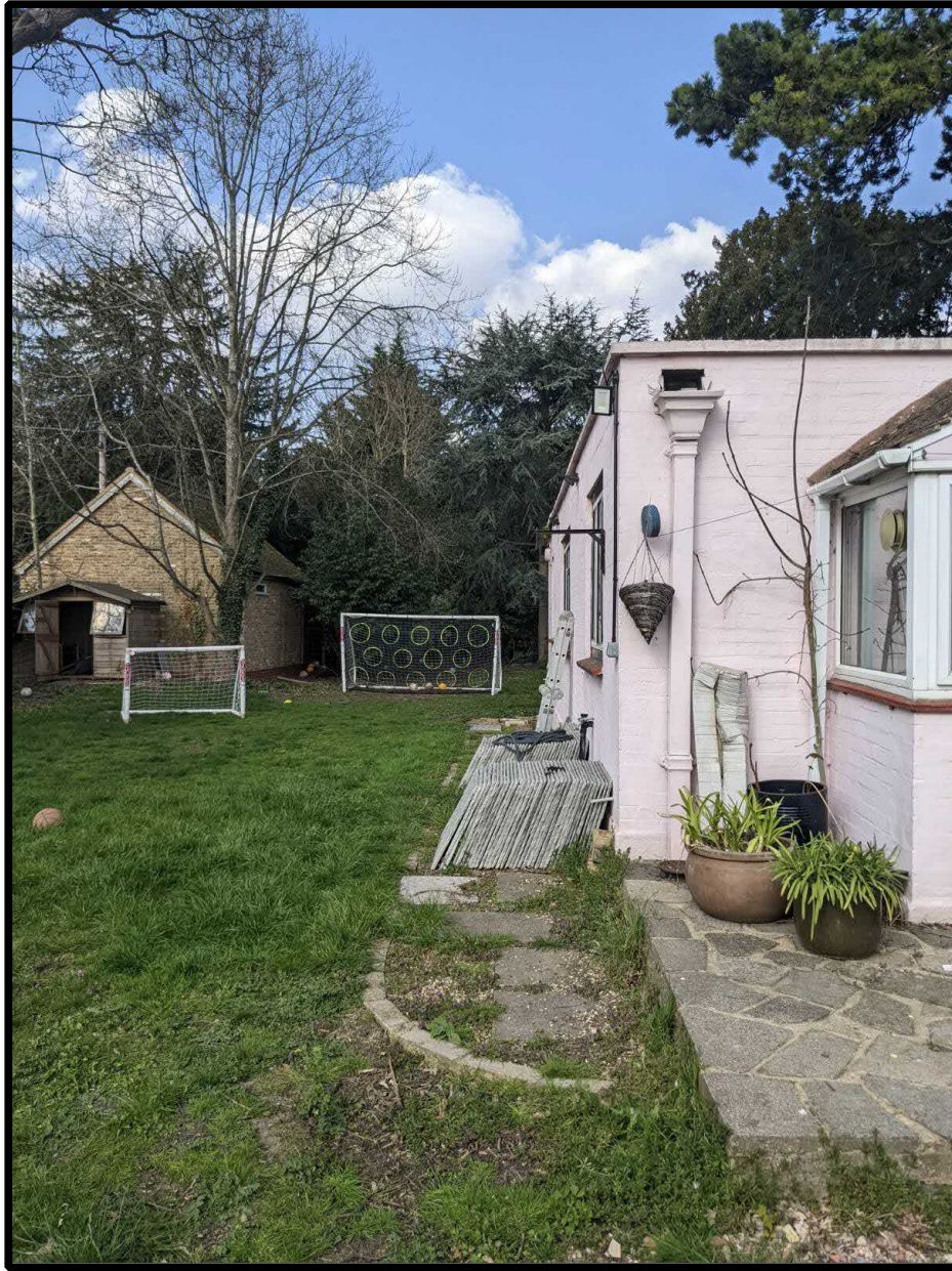
Figure 4 –Photograph of existing rear elevation adjacent to the RPA of T13.
