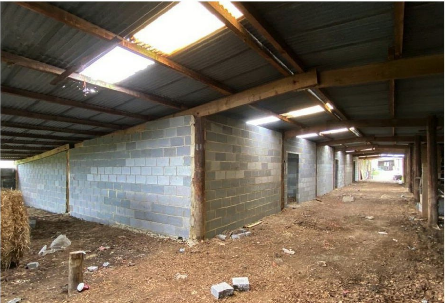
Photo 9. Interior of B3
