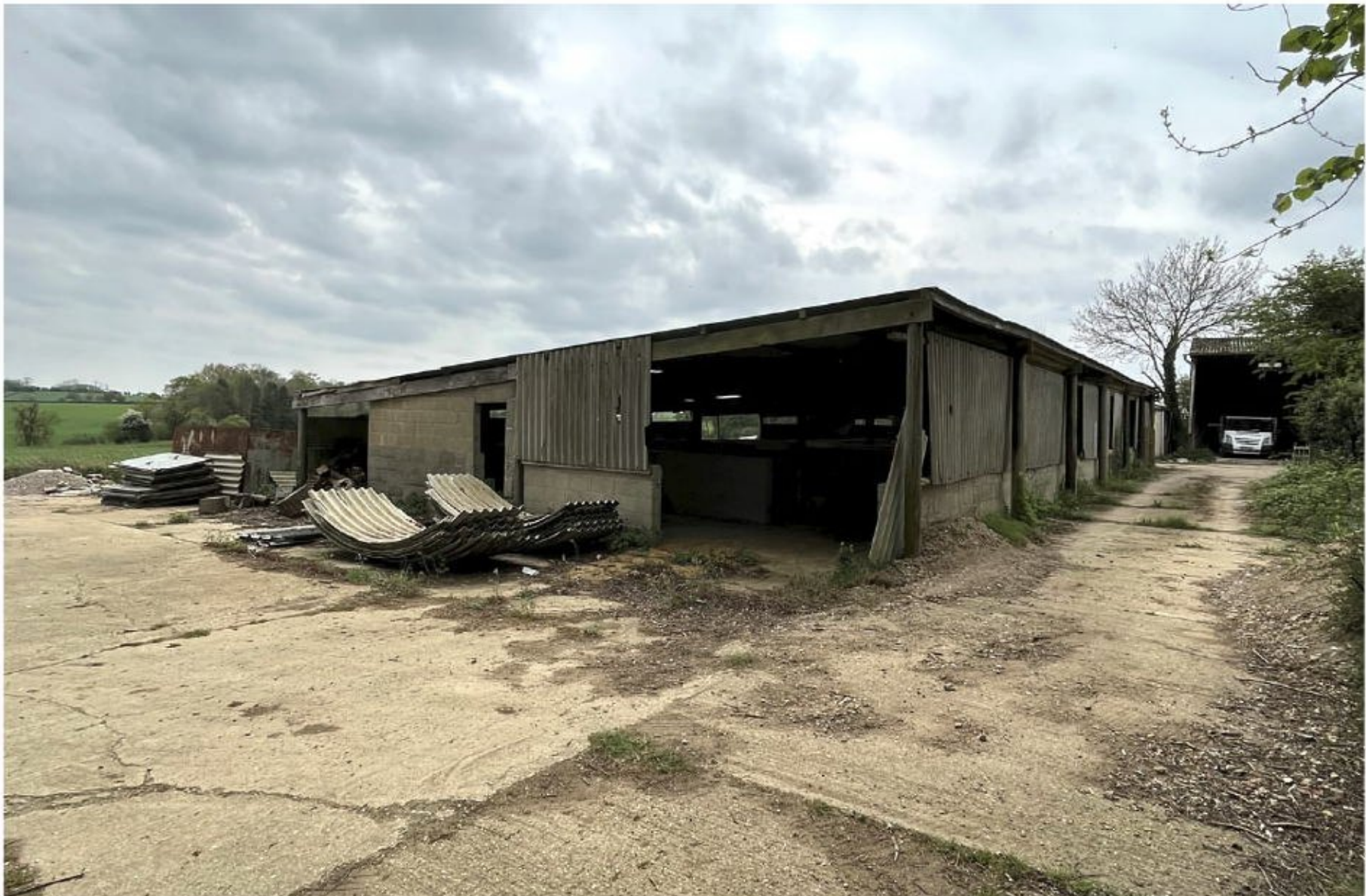
Photo 5. B1 north side, showing surrounding hardstanding
