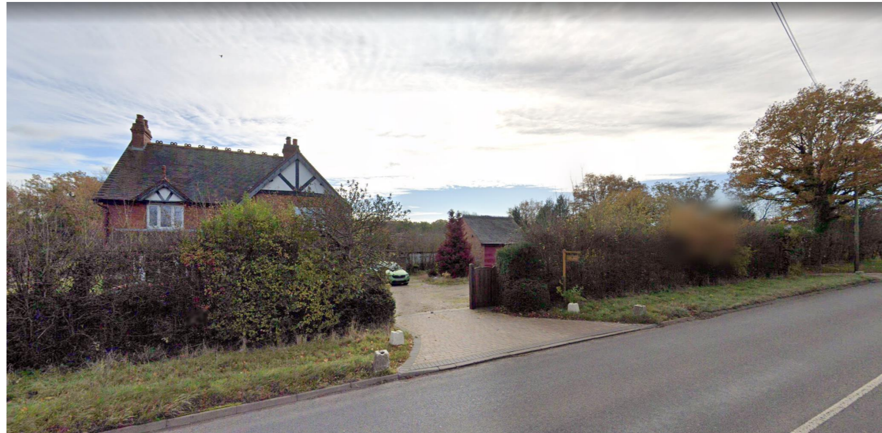
View of existing site entrance from North
