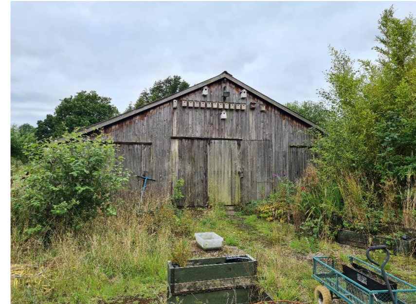
Annex – former piggery
