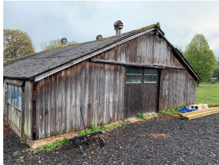
Annex – former piggery
