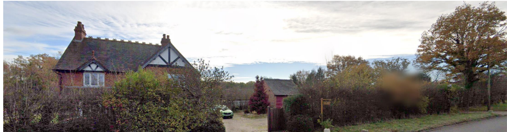
View of application site from the public highway Meer End Road
