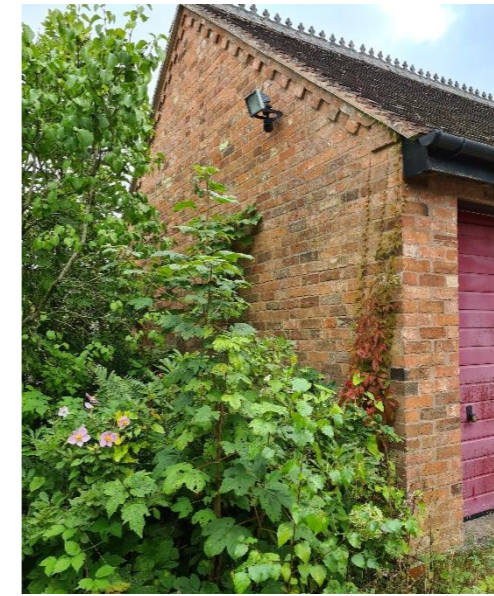
Modern built red brick two car garage
