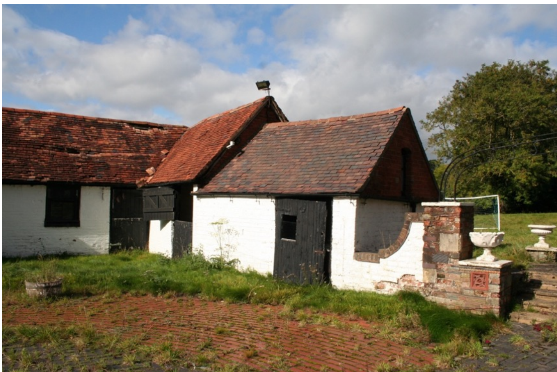
Fig.10 A small addition (right) to the L-shaped range of outbuildings was built in 1917-1925.
