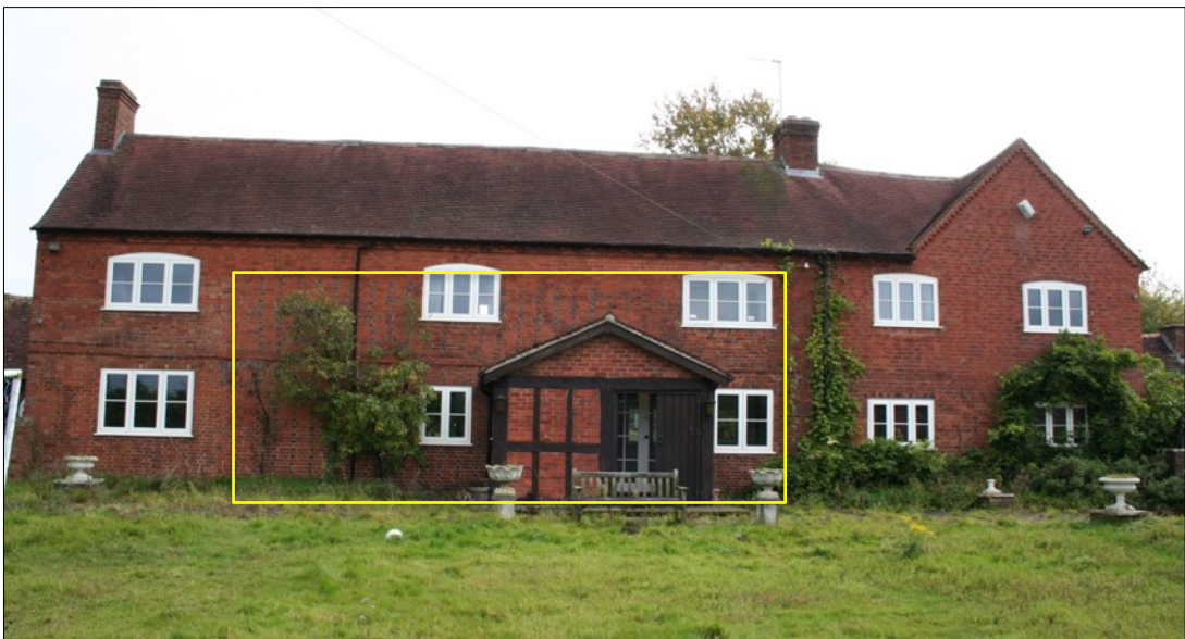
Fig.4 West elevation of Arbour Tree farmhouse indicating the original part of the building (yellow line, excluding the modern porch).
