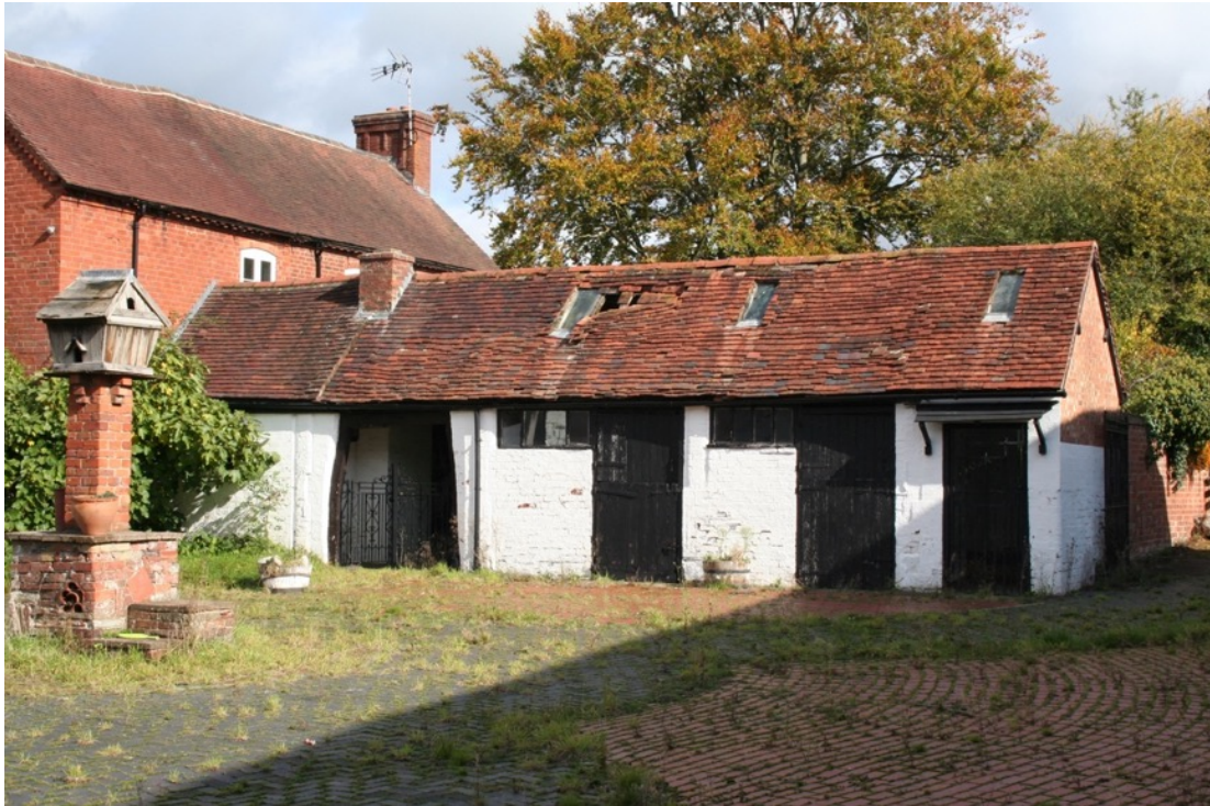
Fig.14 Range of outbuildings adjoining the south of Arbour Tree farmhouse.
