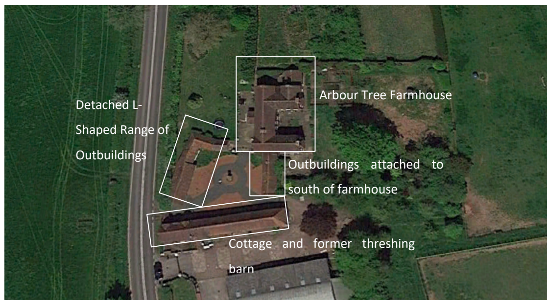
Figure 1 Extant buildings within the application site. Source: Google Earth.
