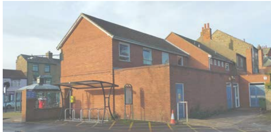
Above: Photo of existing south-east corner of building, taken from car park.
