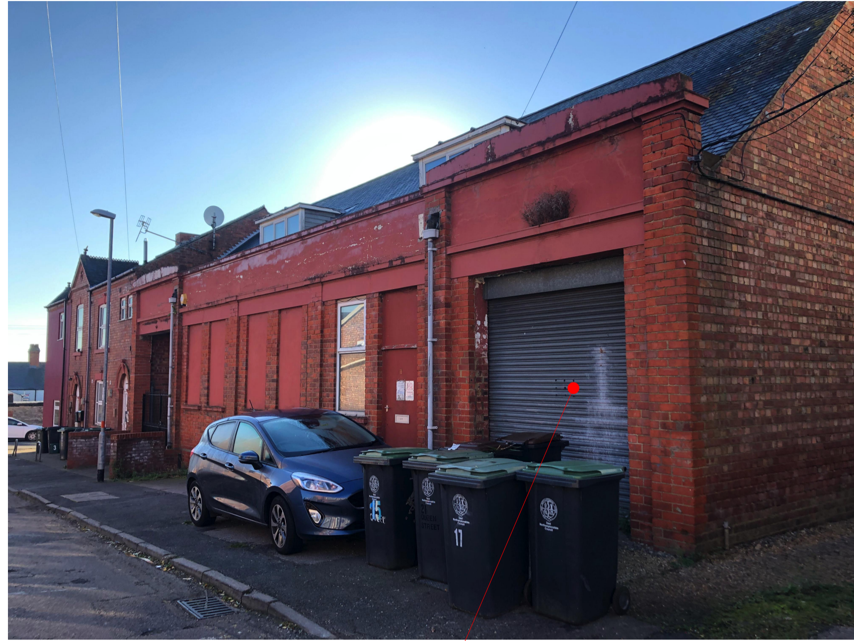
View from Queen Street showing the industrial building adjacent to the rear driveway.
