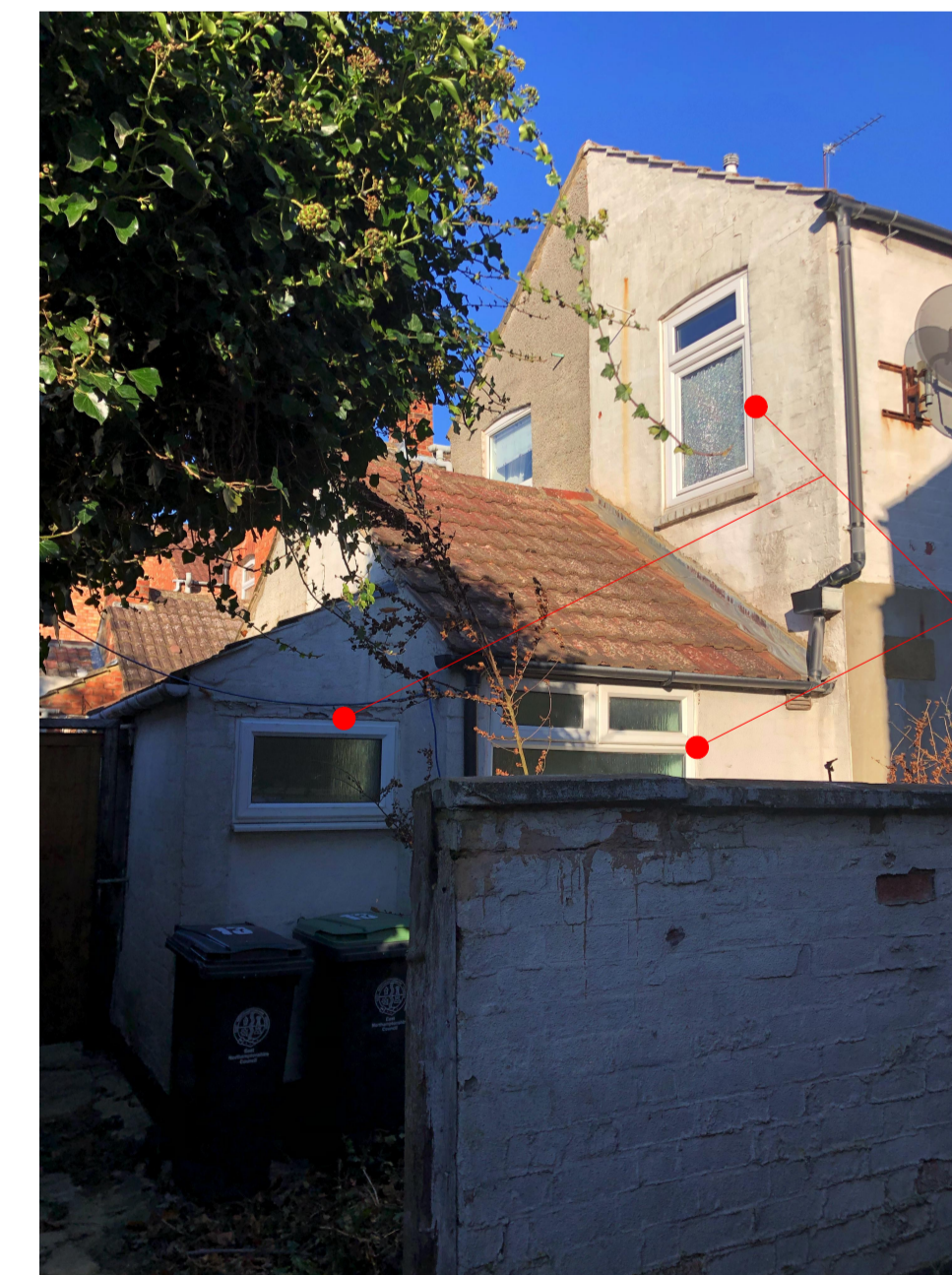
The 3 windows closest to our site (positioned on 13 Queen Street) are from non-habitable rooms and the windows are obscure glazed.
