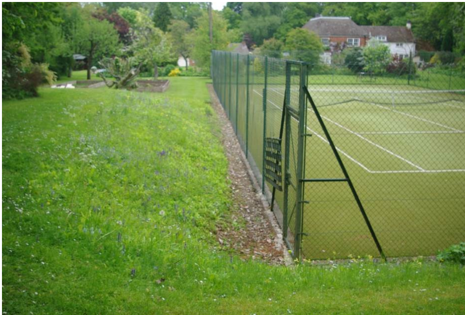
Figure 6. The level reduction west of the tennis court, looking north.
