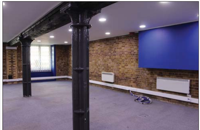
Plate 4. Internal view showing cruciform columns, looking east.
