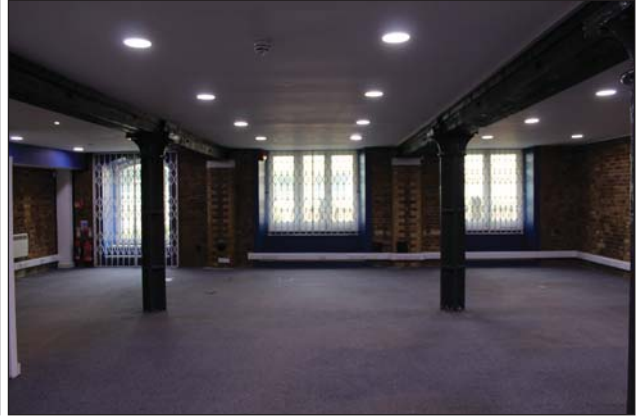
Plate 2. View to windows looking northwest.
