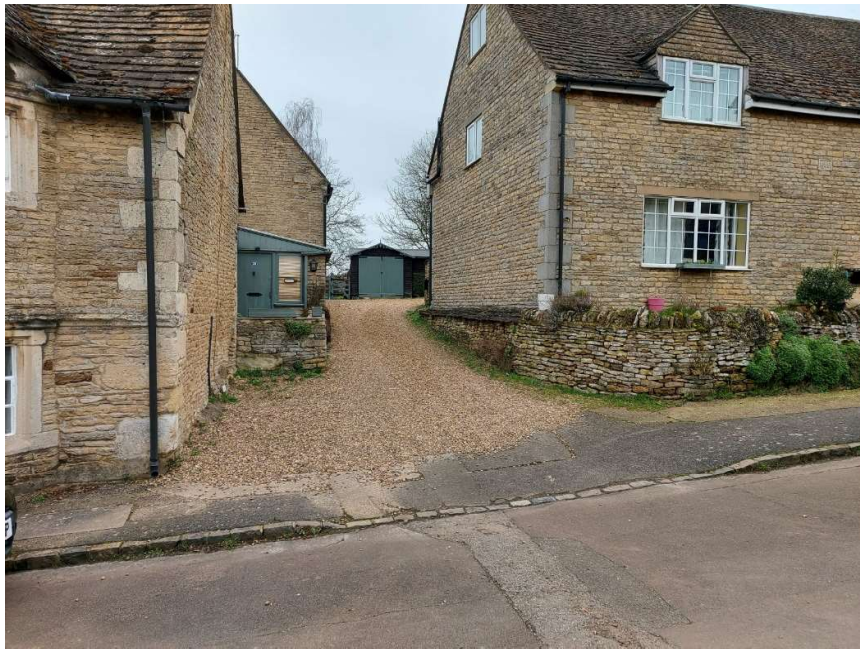
26 High St Three houses share this driveway.
