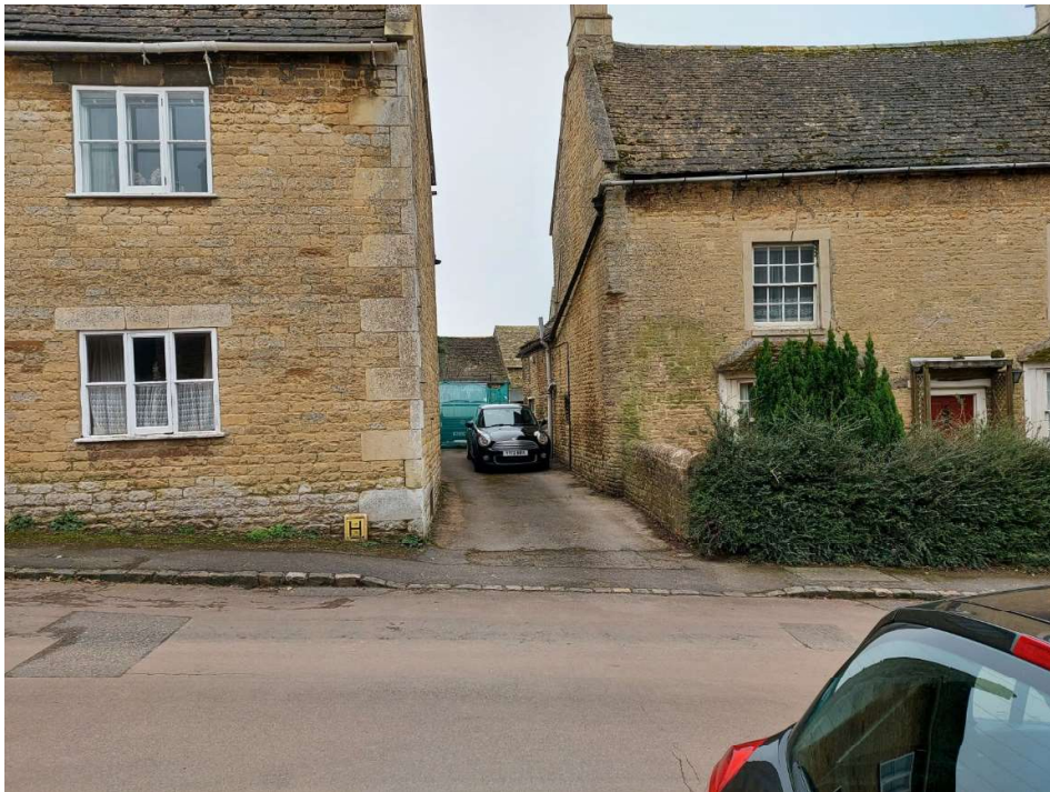
27 High St Two houses share a drive on to the High St. There is no visibility splay at the back of the narrow pavement
