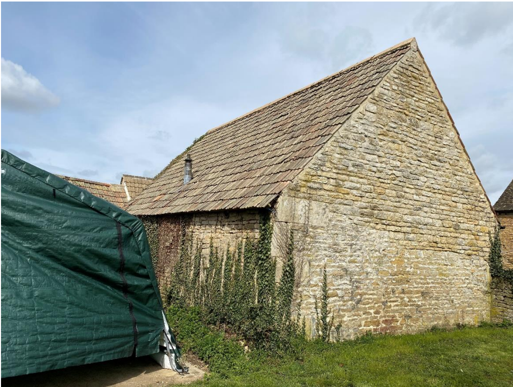
Plate 5 Building 2 - End View
