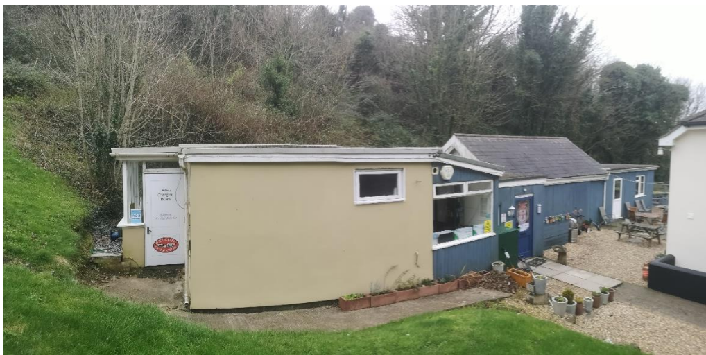
Figure 2. The northern elevations of the Clubhouse
