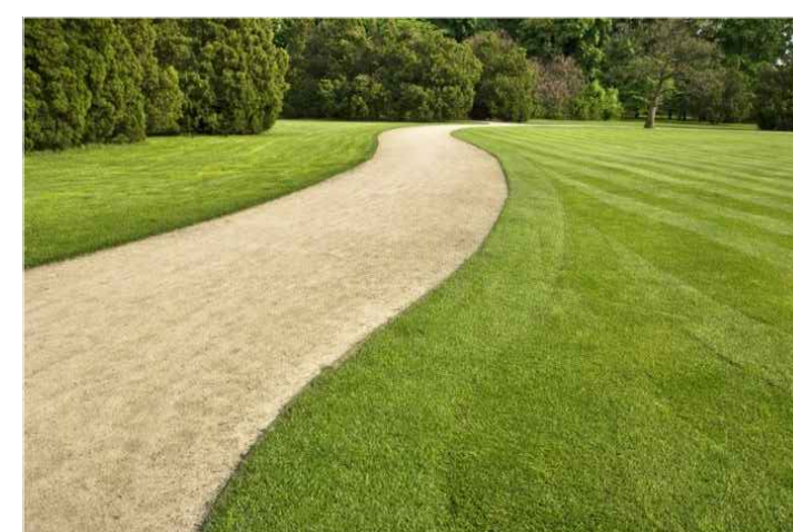
Self-binding gravel surface
