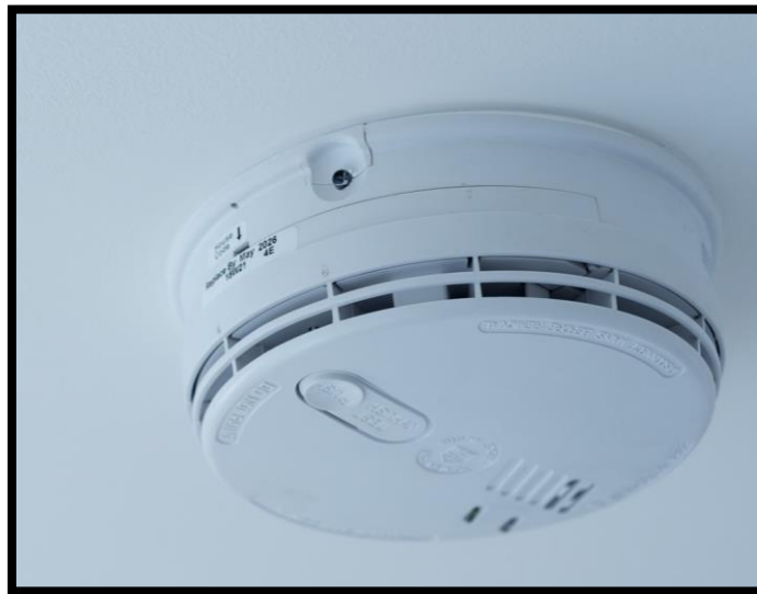
Example of main operated, interlinked fire detector
