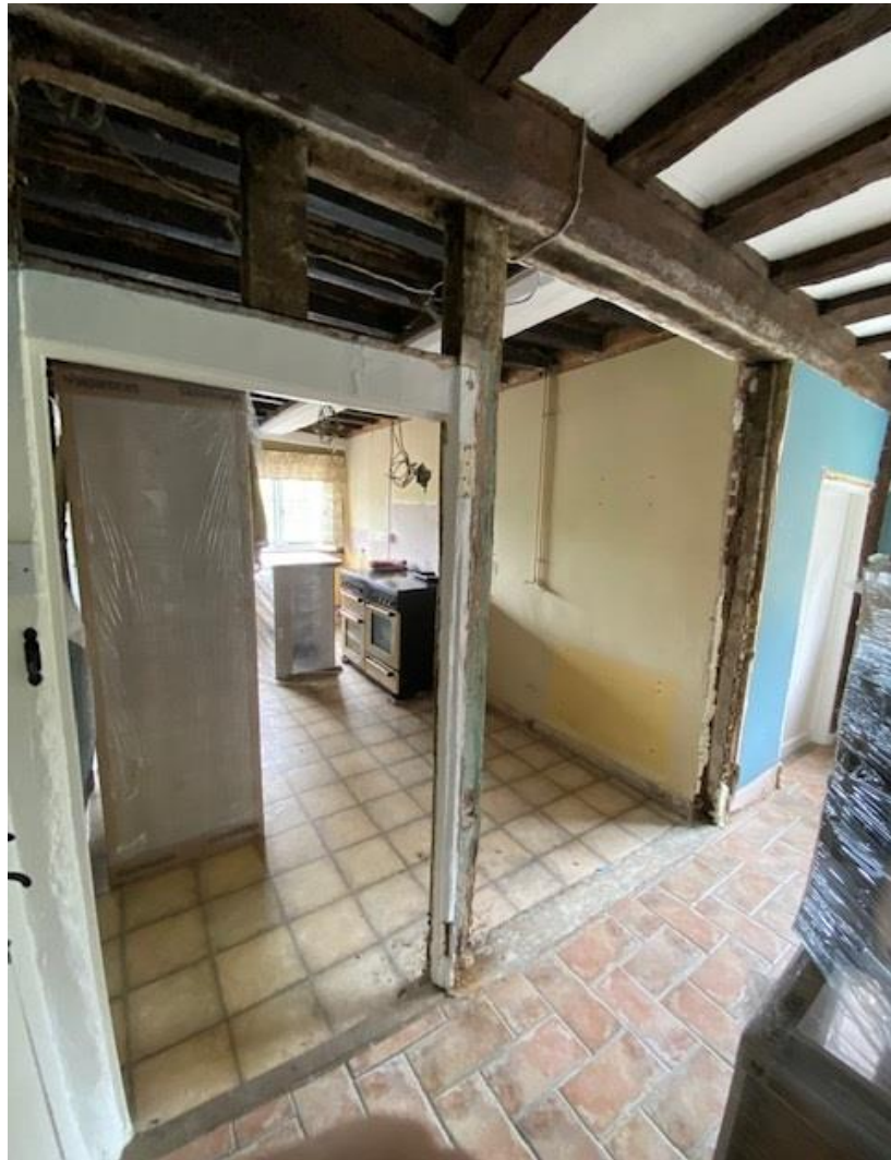
Picture 1. Wall A with the middle section removed which was softwood timber frame studding
