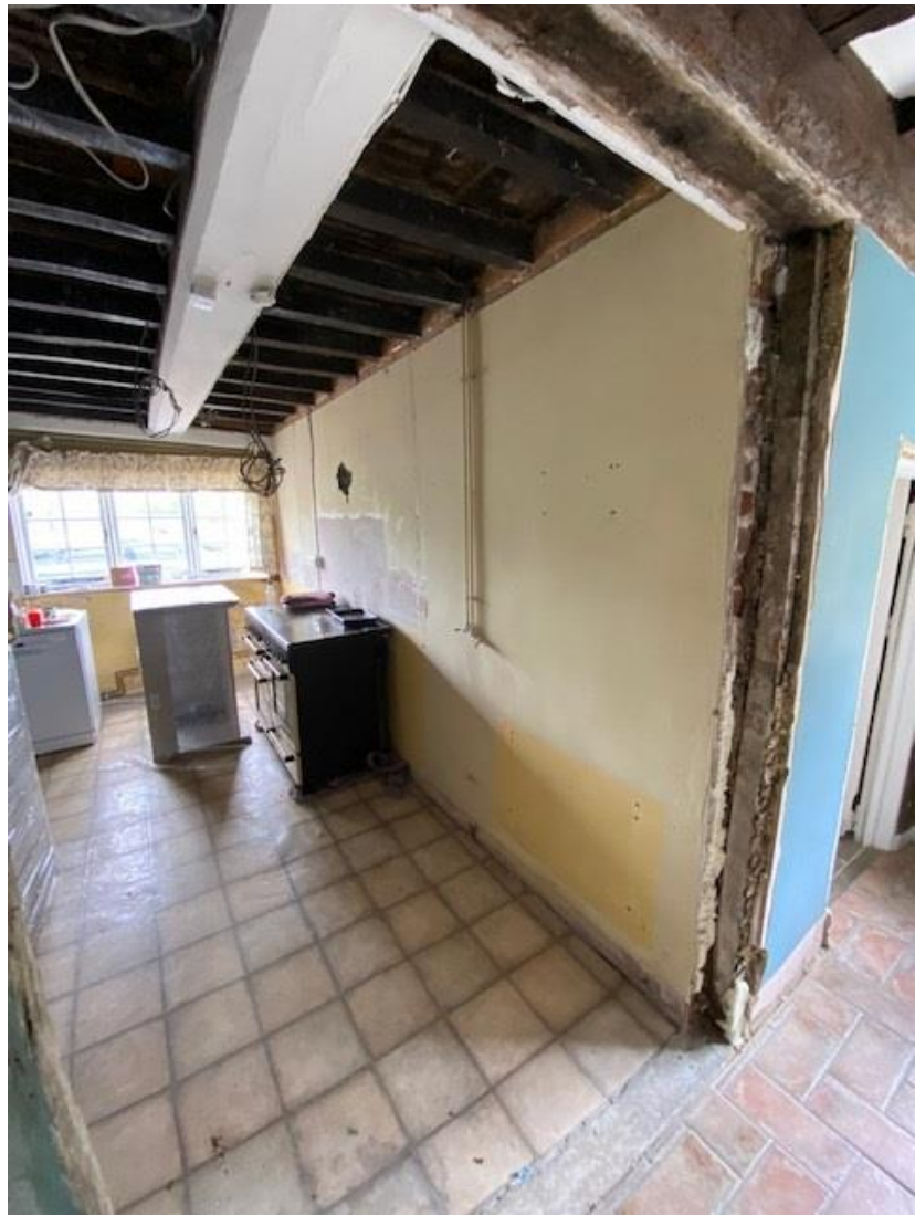
Picture 5. Wall B
