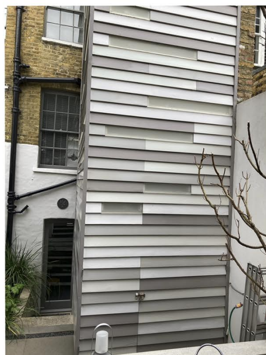
Image 5 - existing rear extension detail
