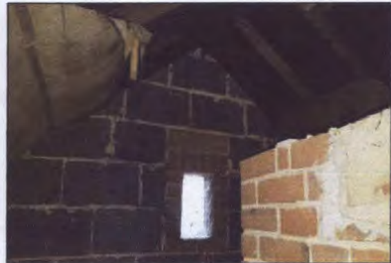
Figure 6: Eastern gable end window.
