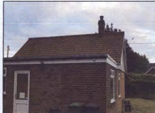
Figure 4: Northern aspect with flat roof extension.
