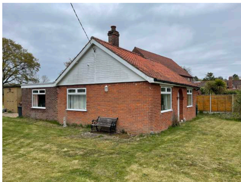
Fig. 1 Existing House Photo
