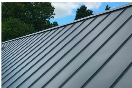
EXAMPLE OF STANDING SEAM ALUMINIUM ROOF
