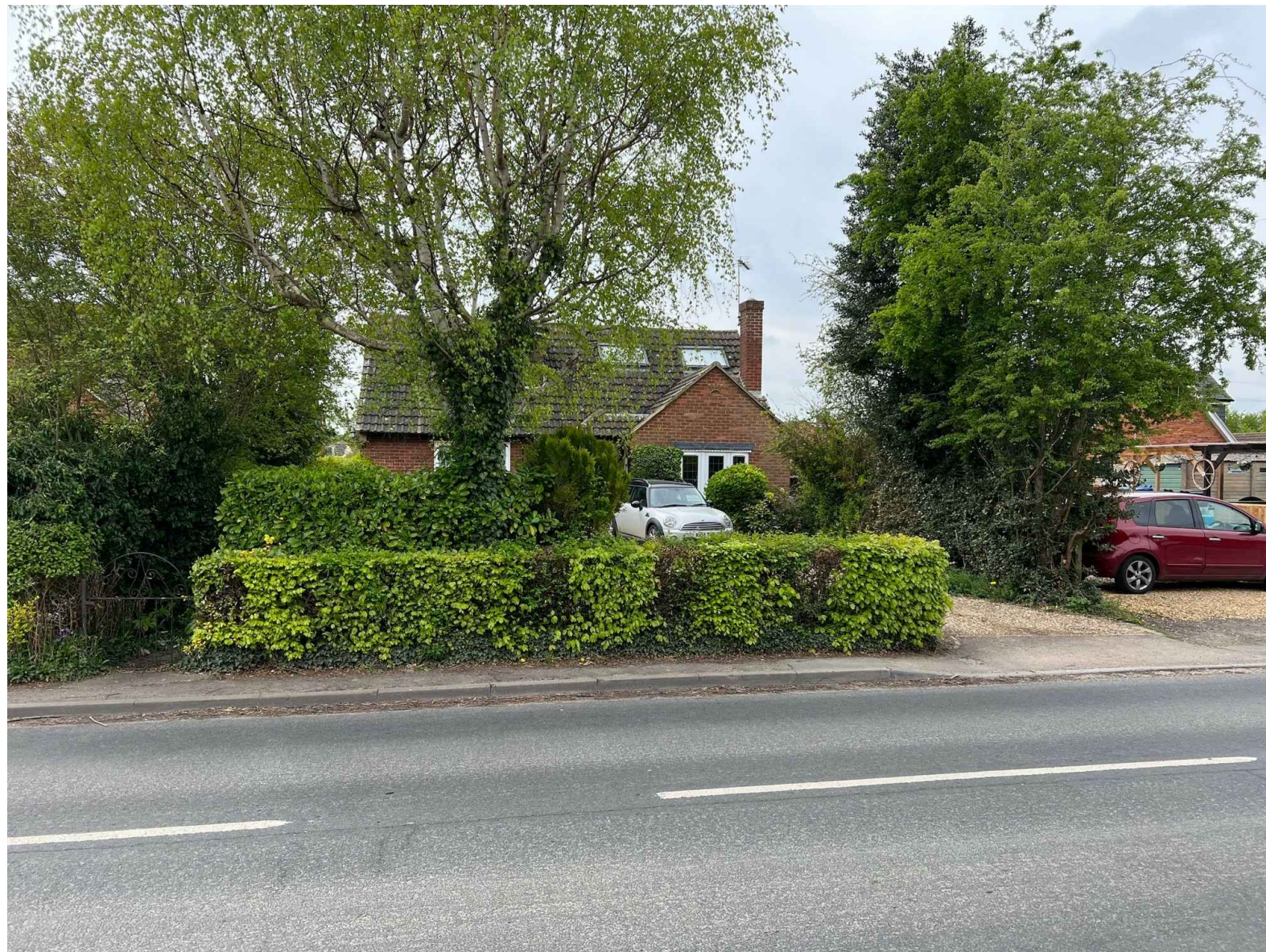
original hedging to back edge of footpath forming visual highway obstruction in terms of depth and height
