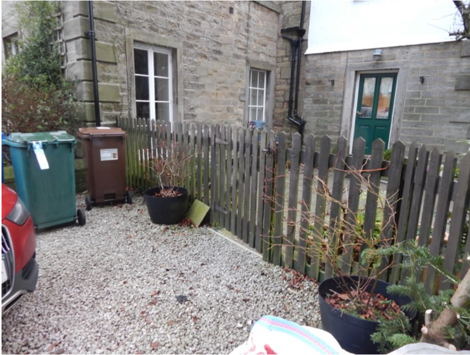
Figure 15 - Existing kitchen entrance and patio / yard
