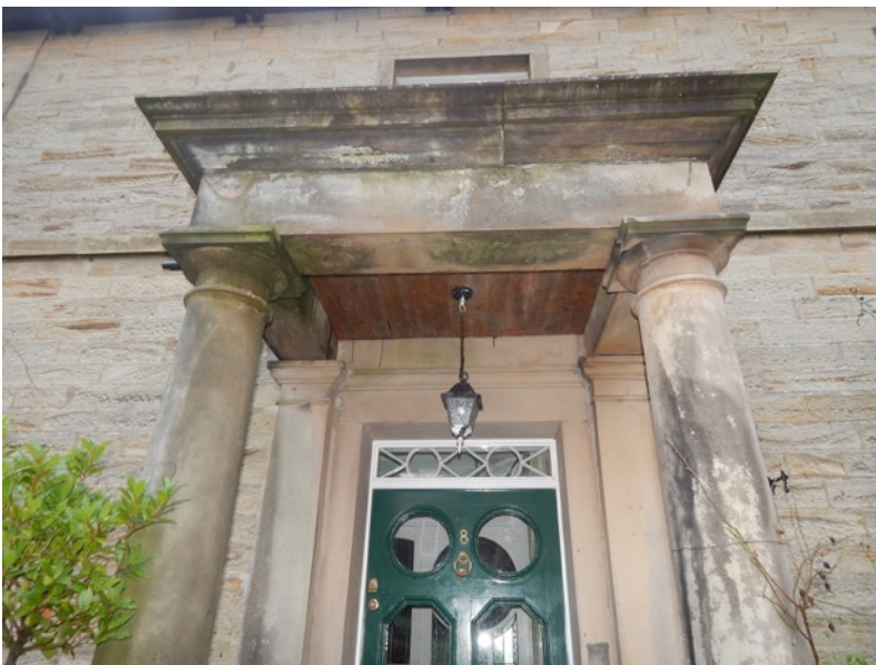
Figure 14 - Existing front porch
