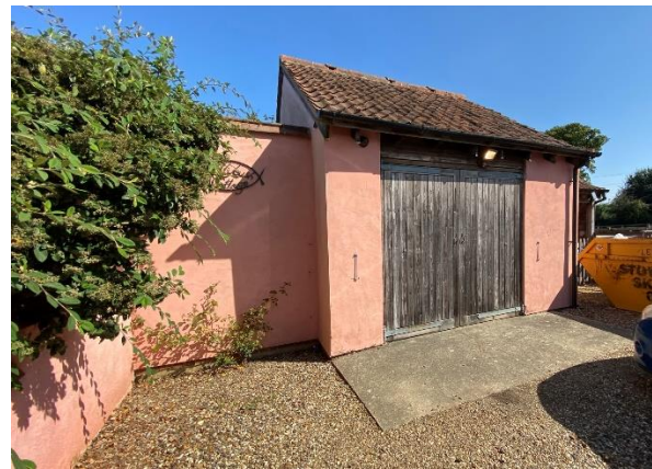
Garage with storage room beyond wall
