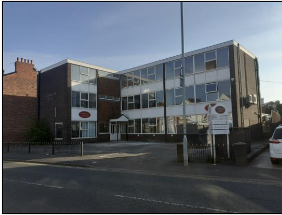
Figure 2: View of Carrwood House from Shaw Heath.
