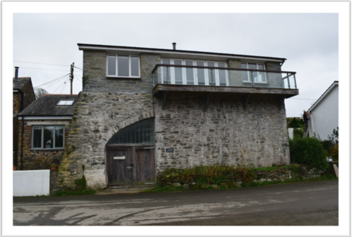
Figure 13 – above, The Old Lime Kiln, Unnamed Road.
