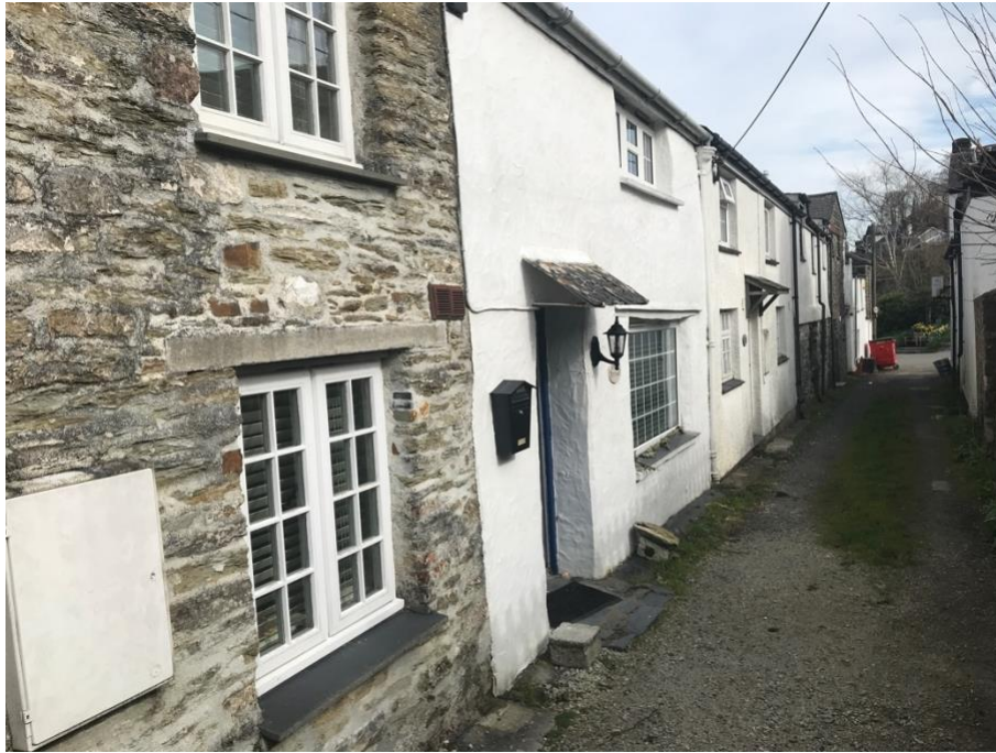
Rear elevation from lane
