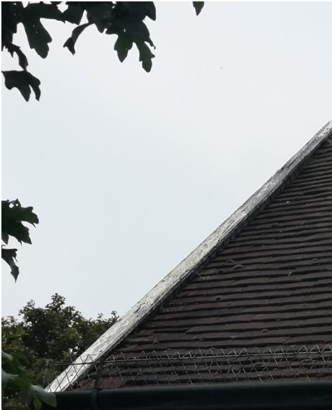
Worn Out woodwork on Roof
