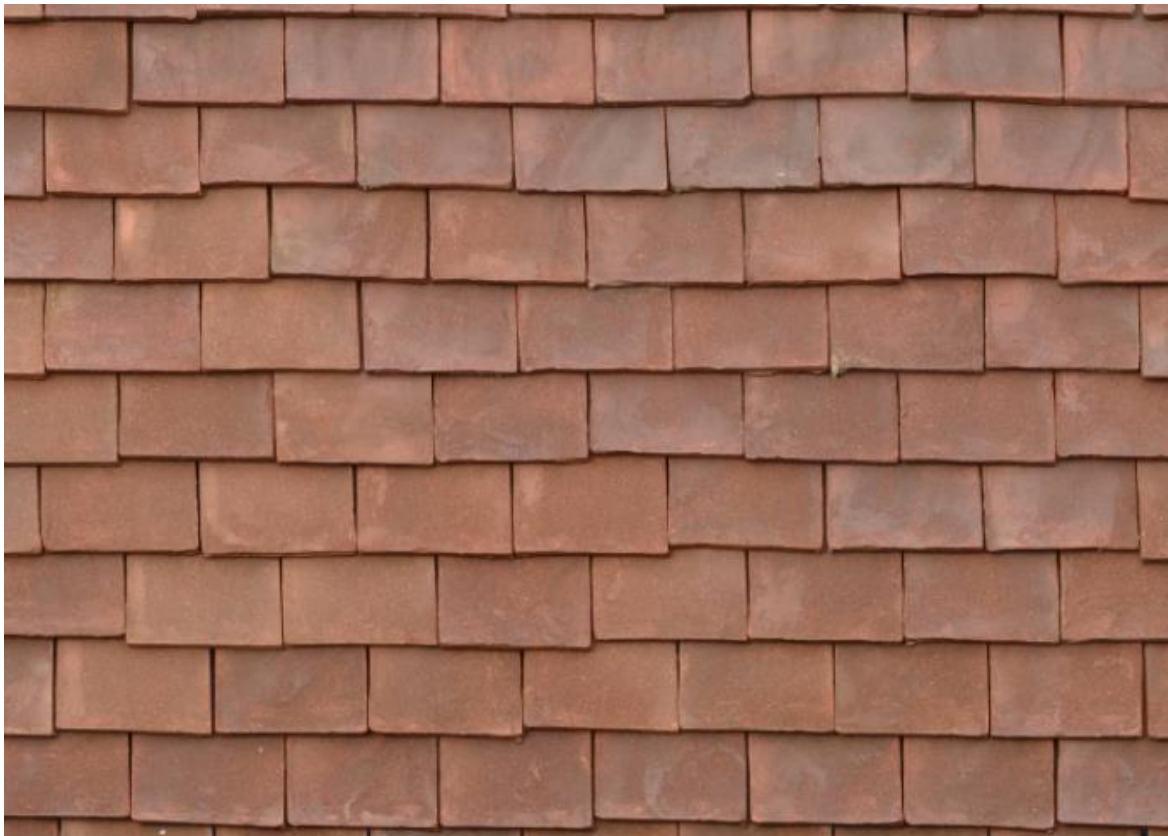
Main Roof Clay hand made plain tiles – Brookhurst
