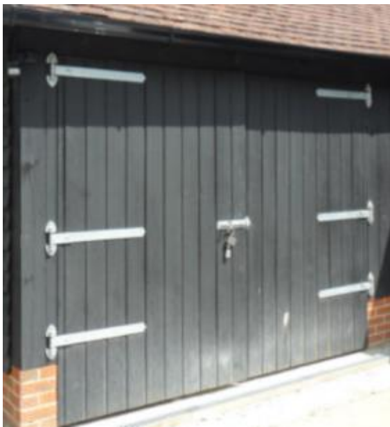
Doors Timber boarded side hung doors
