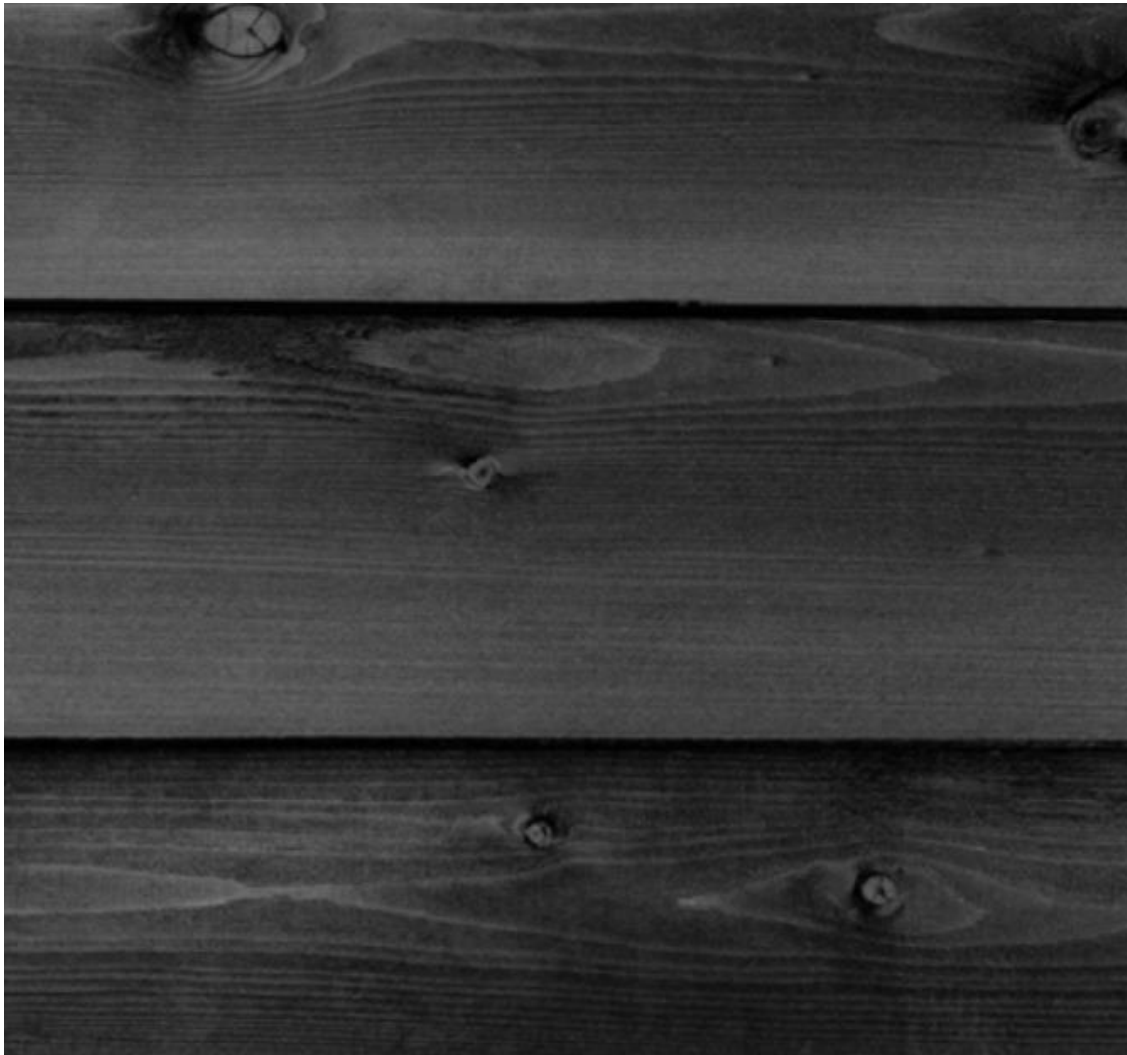
External Walls – Black Timber weatherboards
