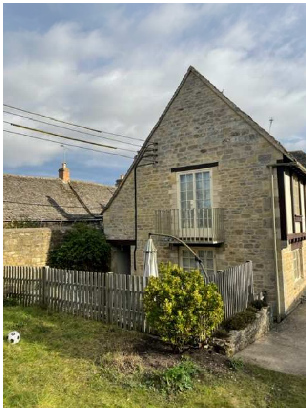
Figure 2 Image of the rear elevation of the 1980s extension
