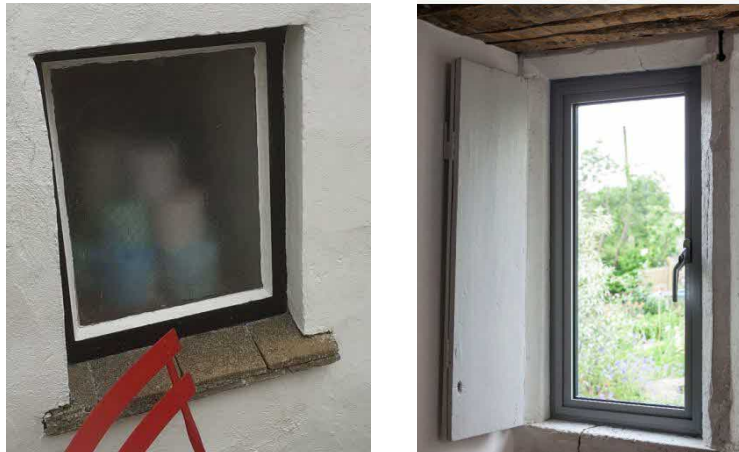
The current window and tile sill left, and an example of a simple Alitherm Heritage window right.
