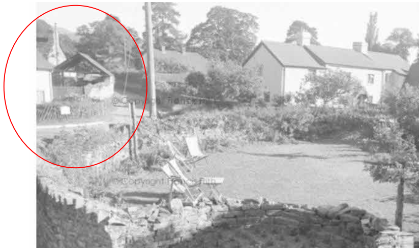
1950 photograph showing the south west corner of Lamb House with the outbuilding behind that appears as an open shelter shed at this time without cladding.
