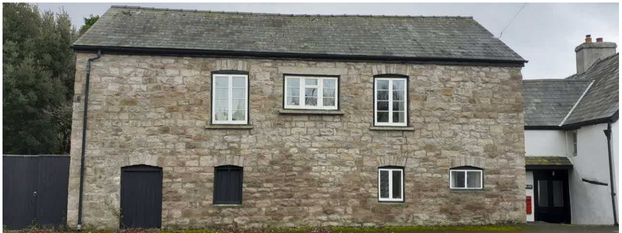
The north elevation of the barn
