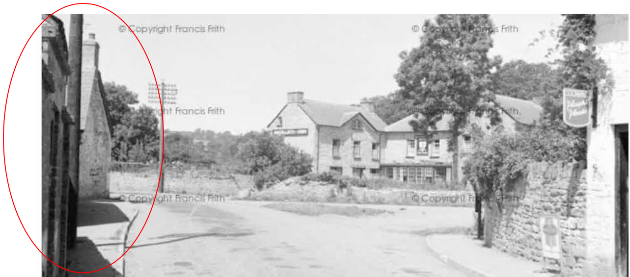
1957 photograph showing the roadside gable of Lamb House with a 'bagged' /'parged' finish.
