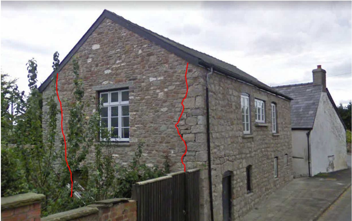
Google Street view showing the re-built gable of the barn between the red lines.
