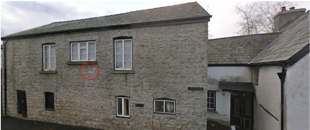
Google Street View 2009 showing the cement slurry finish on the barn although elements of limewash do survive (circled)
