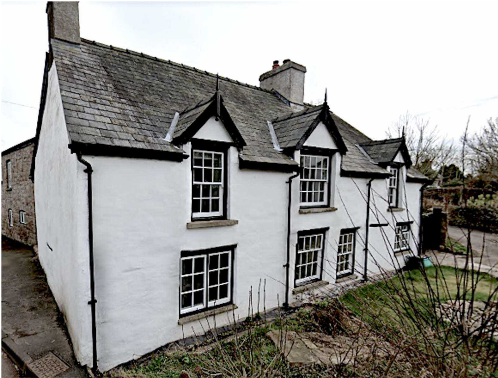
Alterations and Renovations at Lamb House, Glasbury
