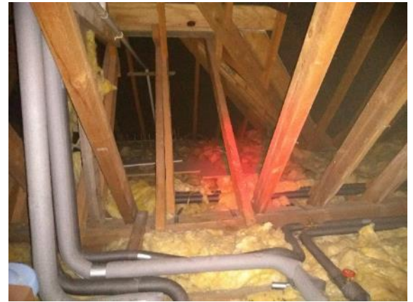
Photograph 4. Loft space north of attic room
