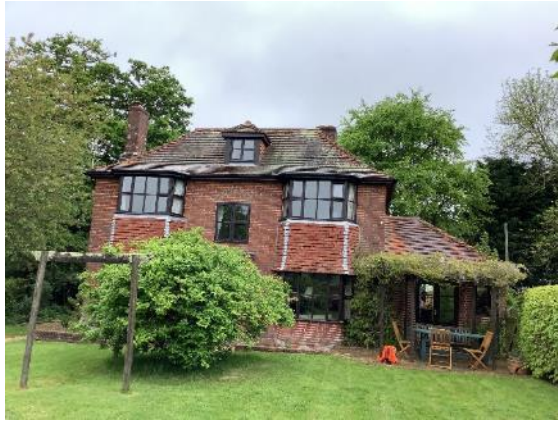
Photograph 1. South aspect of residential dwelling showing single dormer window of attic room
