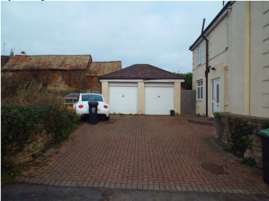
Garage to be demolished
