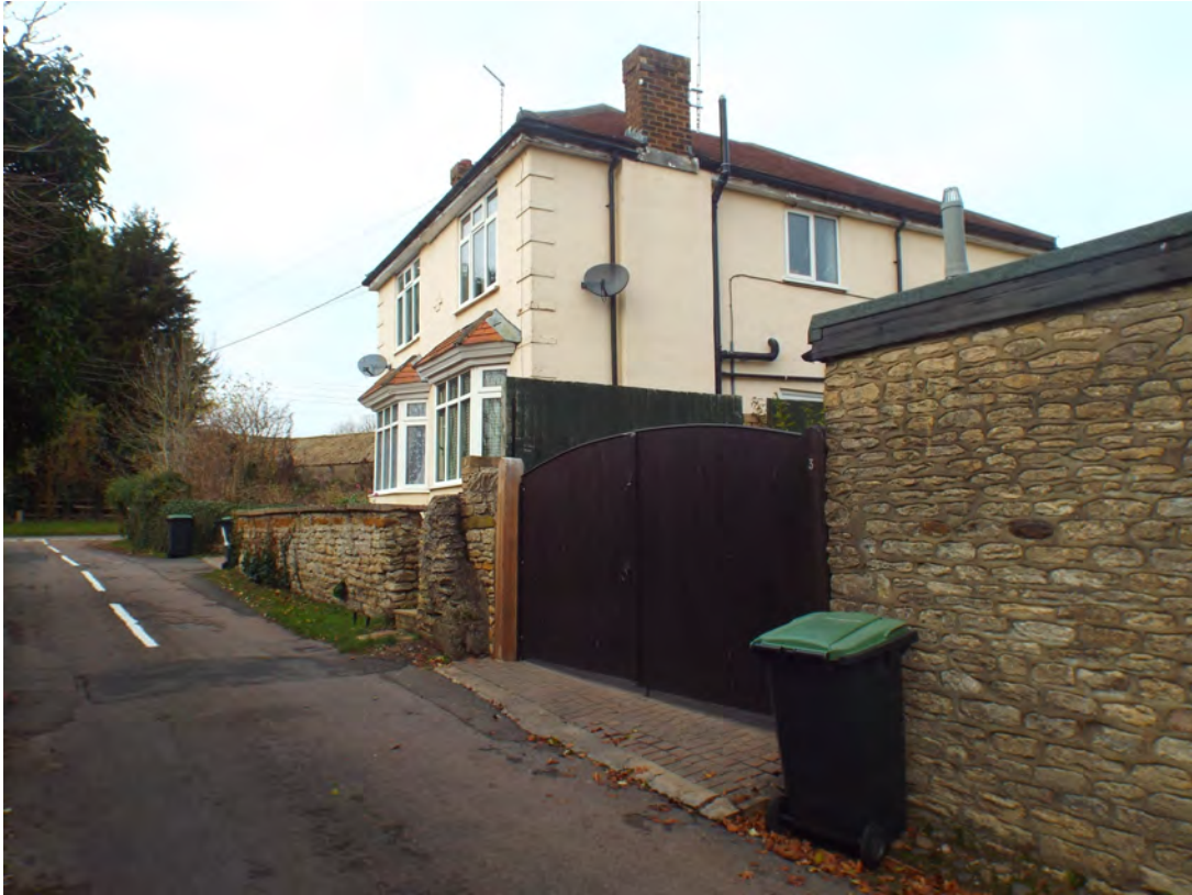
1 and 1A Rectory Lane
