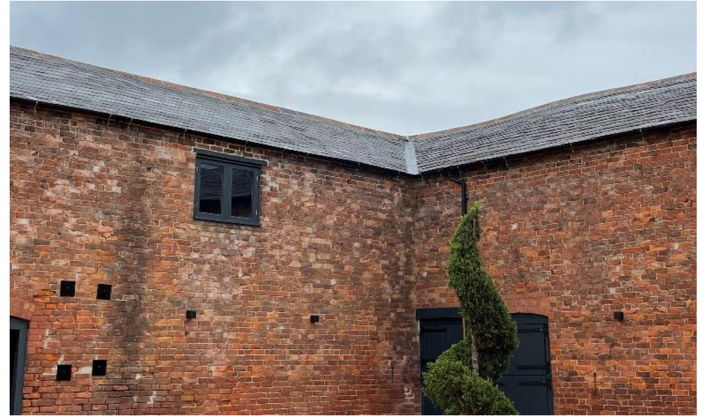
Example of the current exterior roof structure of B1 (pictured above).
