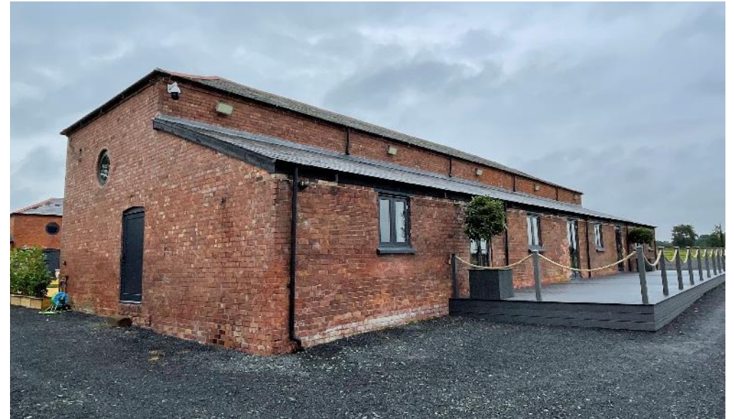
Eastern elevation of B1 (pictured above).
