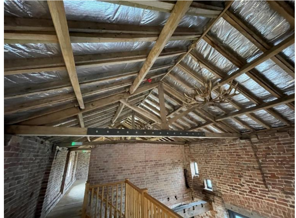
Western internal section of B1 (pictured above).
