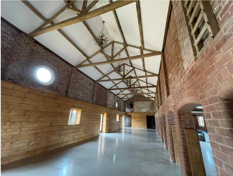
Eastern internal section of B1 (pictured above).
