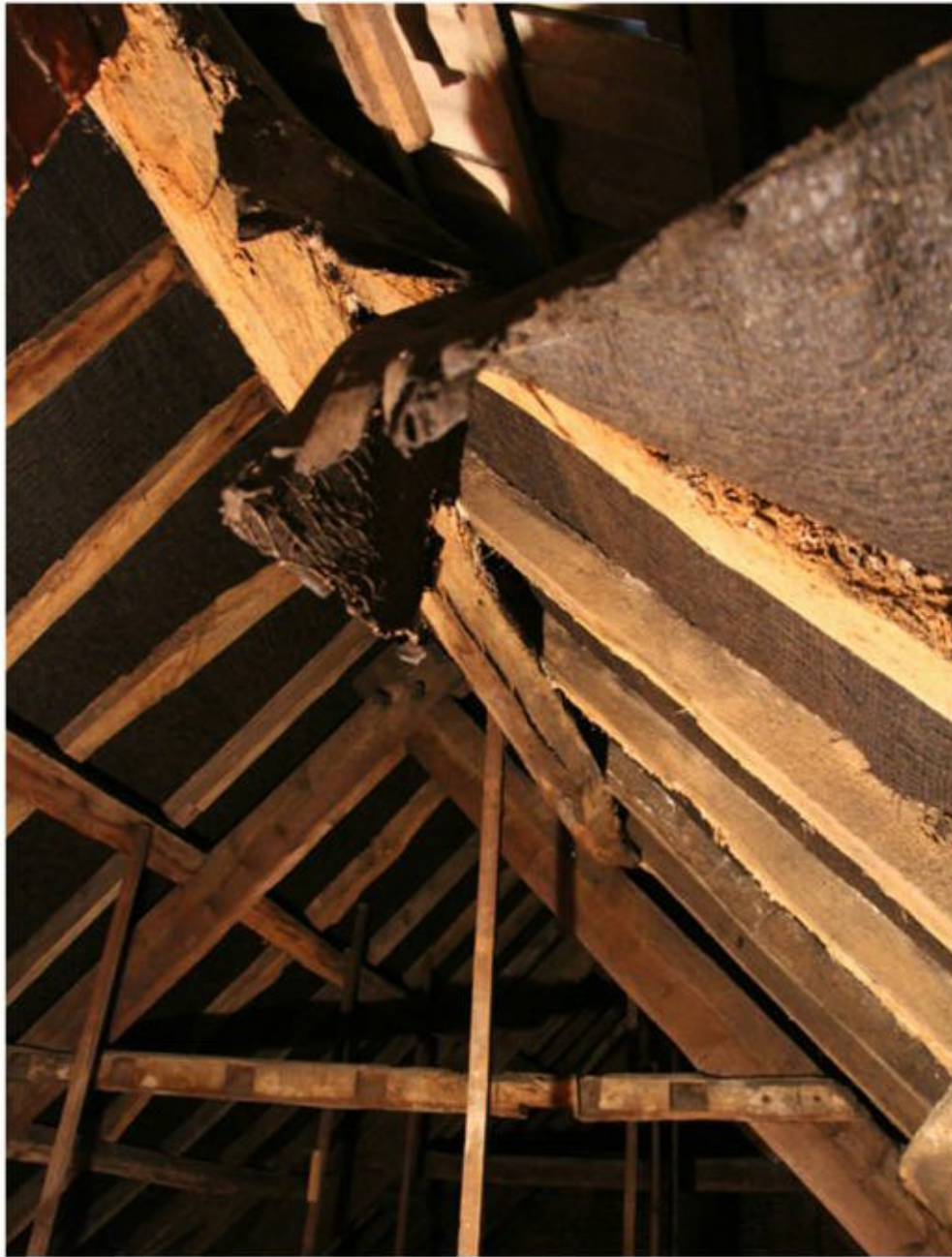
Image 4: Main Roof Internal View
