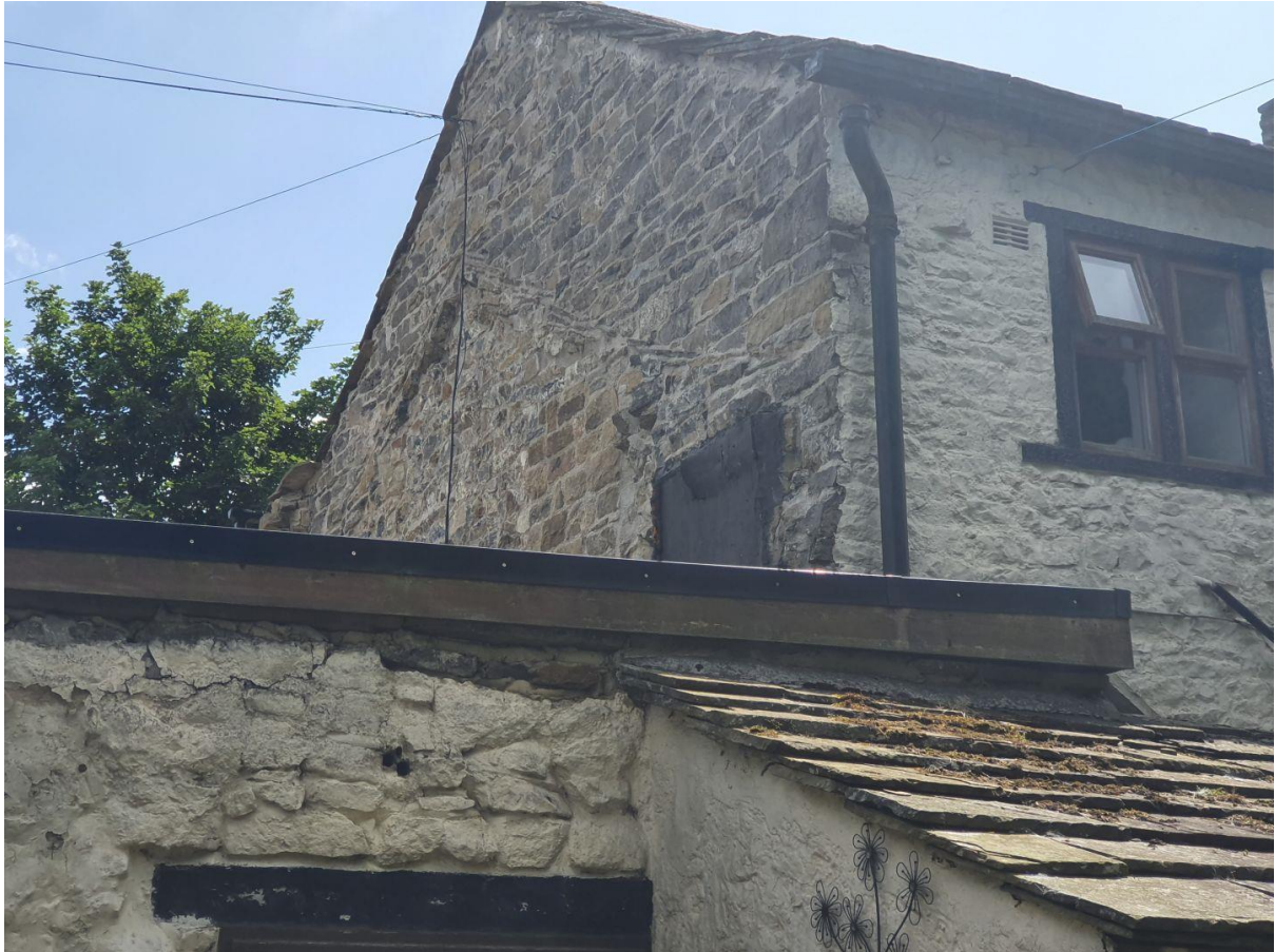
Closer view looking towards North Elevation
