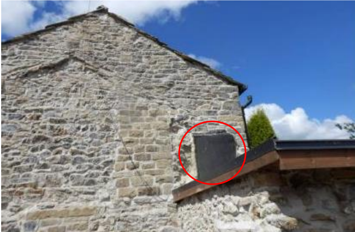
Image 3 View of infilled hole in the party wall when exposed following demolition of Nuttercote Farm.
