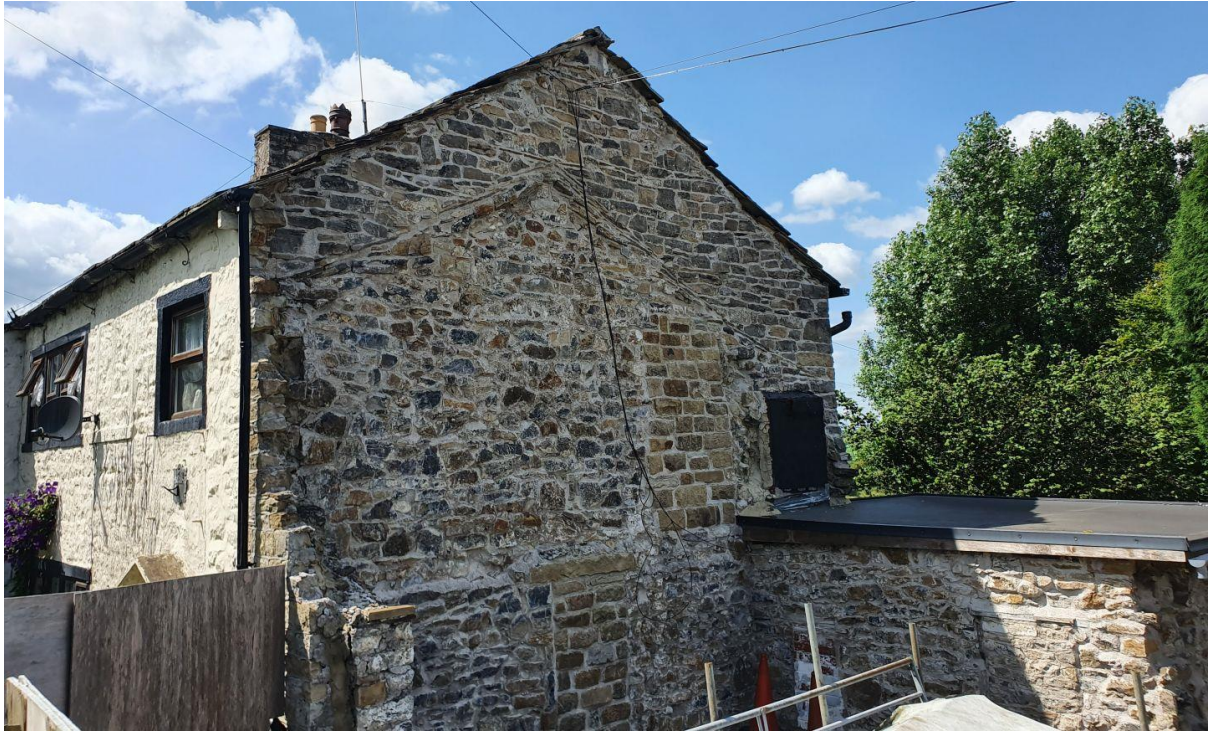
View looking towards gable elevation (East Elevation)
